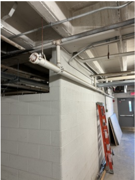
Picture indicating routing of Geo Thermal Conduits in the Basement Level.
