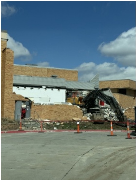
Peitzmeier Demolition used to back hoes to take down the roof structure of the Blue Gym. Picture taken on 4/3. They are hauling out the separated concrete and steel daily as the take the building down.
