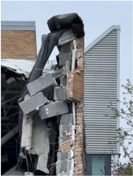
Typical wall section of the old Blue Gym had foam insulation in the cavity between the CMU wall and the Brick veneer.
