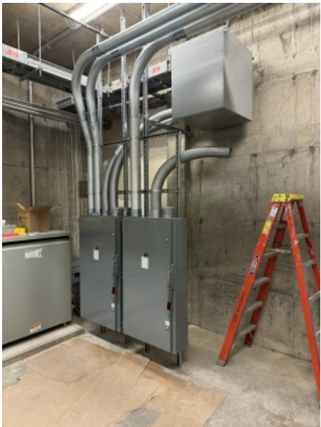
Part of getting the pool building ready for demo is the refeeding of the power serving the Geo Thermal Heat Pump Loop pumps and misc mechanical equipment. This picture is in one of the main Electrical Rooms near the main Gym. One temporary disconnect is for the Heat Pump Loop, and the other is for a new panel on 2nd floor by Tim's office.
