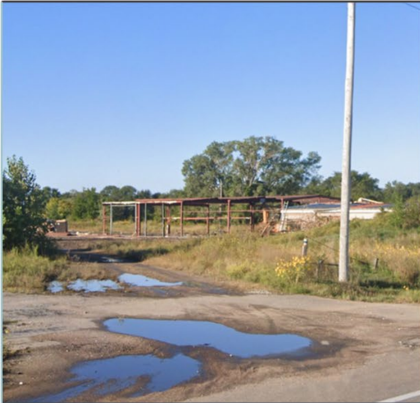
Post Flood Condition
