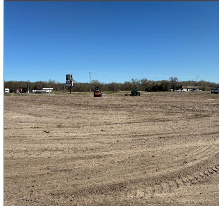
Current - Structures & debris have been removed.
