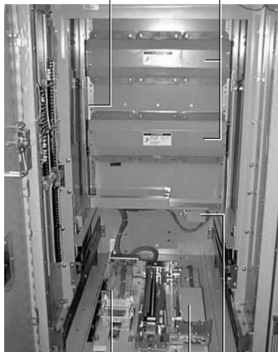
38 kV Switchgear—Control Compartment
