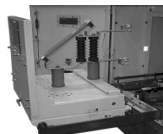
Fuse Drawer—Shown Fully Withdrawn
