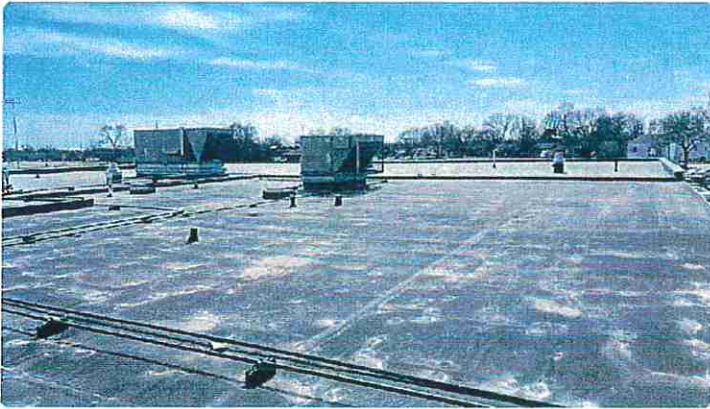
Photo showing an overview of the High School section roof.
