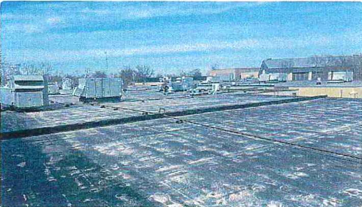
Photo showing an additional overview of the High School section roof.
