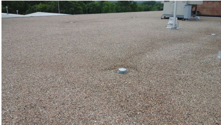
Photo showing overview of Area 06 Roof.
