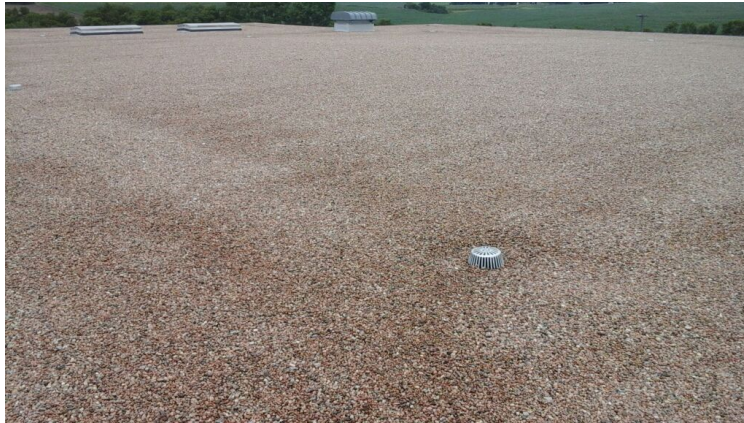
Photo showing overview of Area 07 Roof.
