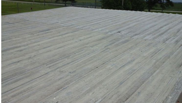
Photo showing overview of Area 04 Roof.
