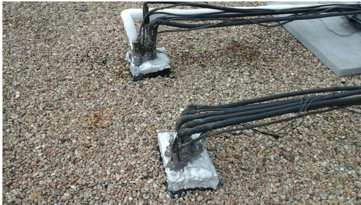
Photo showing condition of the pitch pans.
