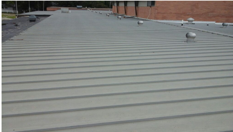
Photo showing overview of Area 02 Roof.
