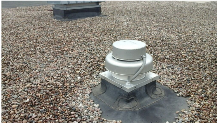
Photo showing condition of projection flashings.
