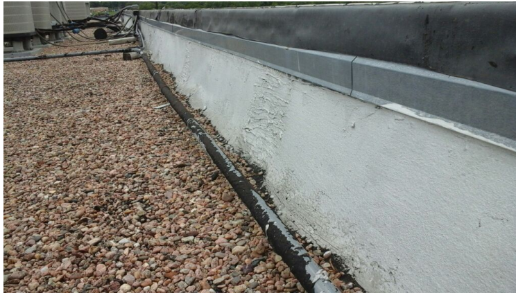
Additional photo showing condition of the perimeter flashings.
