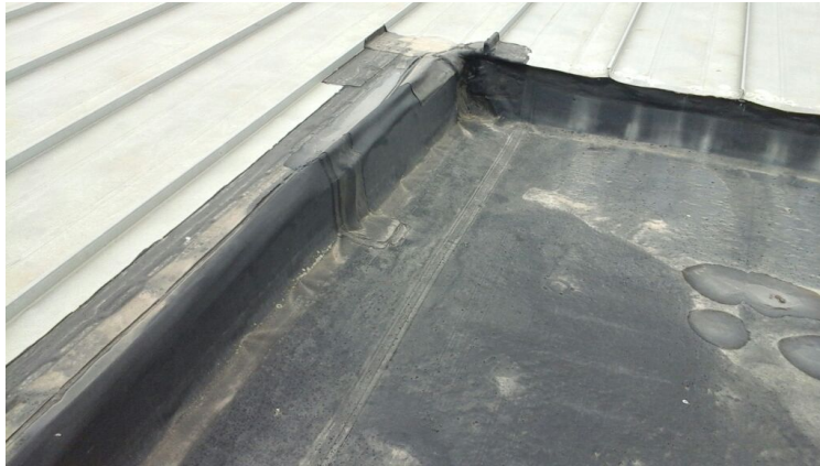
Photo showing connection to adjacent metal roof.
