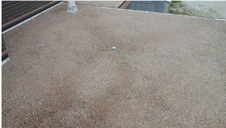
Photo showing overview of Area 09 Roof.
