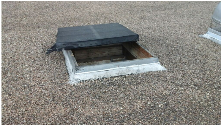
Photo showing condition of the roof hatch.
