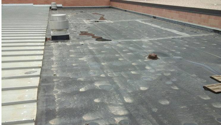
Photo showing overview of Area 05 Roof.
