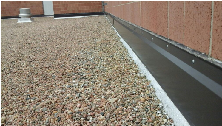
Photo showing condition of the perimeter flashings.
