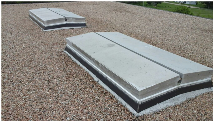
Photo showing condition of stage fire dampers.
