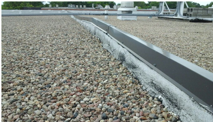
Photo showing condition of flashings along the expansion joint.
