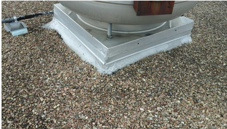
Photo showing condition of projection flashings.
