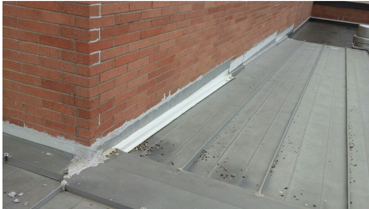
Photo showing condition of the perimeter flashings.
