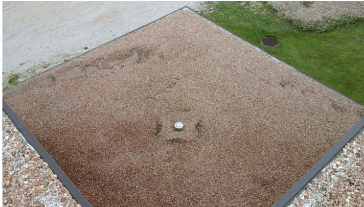
Photo showing overview of Area 08 Roof.
