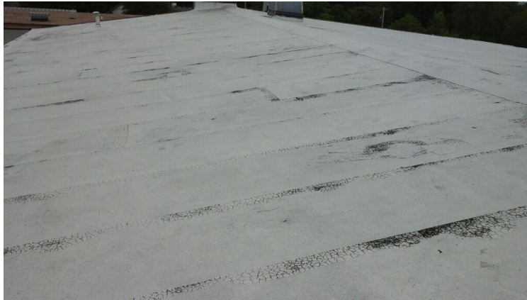
Photo showing overview of Area 10 Roof.
