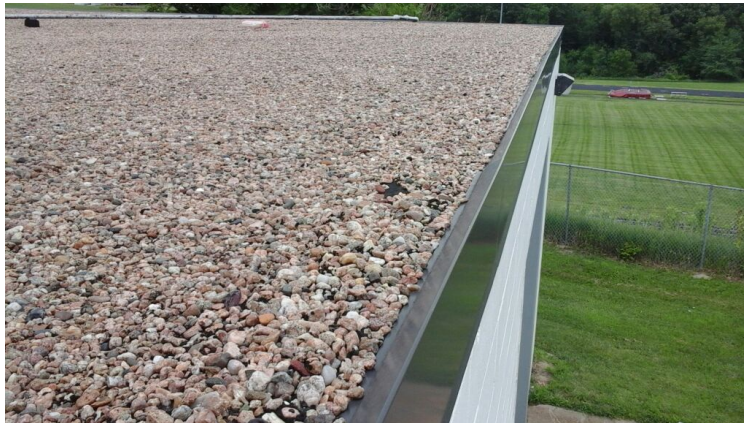
Photo showing condition of the perimeter metal.
