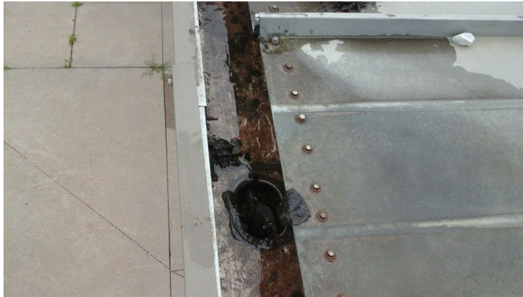
Photo showing drain unclogged.
