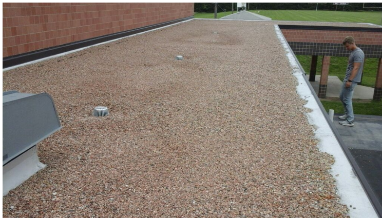
Photo showing additional overview of Area 06 Roof.
