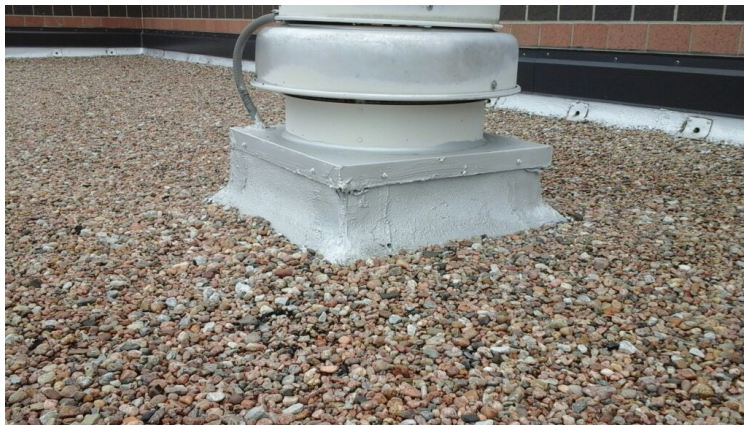
Photo showing condition of projection flashings.
