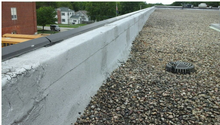
Photo showing condition of the perimeter flashings.
