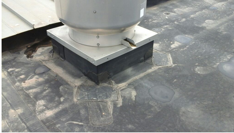
Photo showing condition of projection flashings.
