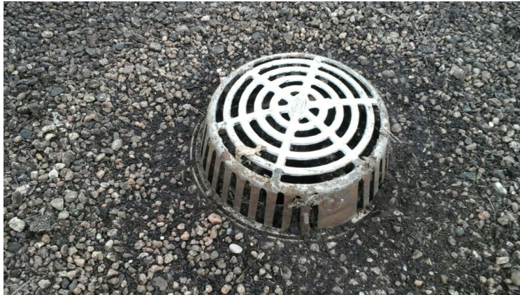
Photo showing cleared drain.
