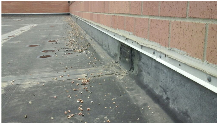
Photo showing condition of the perimeter flashings.
