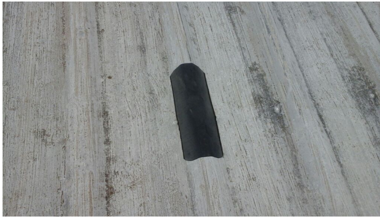
Photo showing a rubber patch on top of coated metal.
