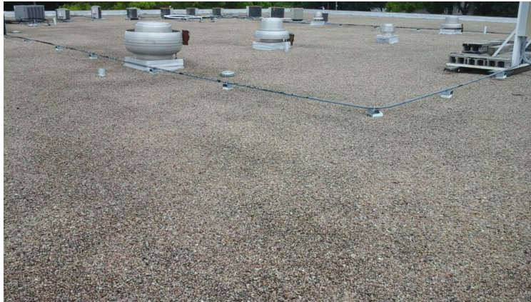
Photo showing overview of Area 02 Roof.
