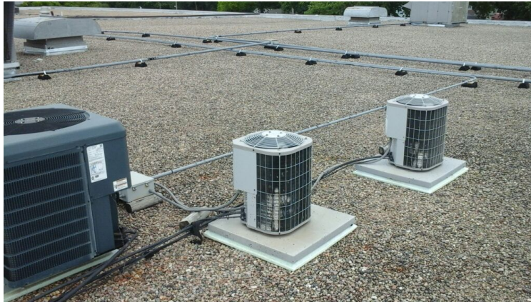
Photo showing overview of Area 01 Roof.
