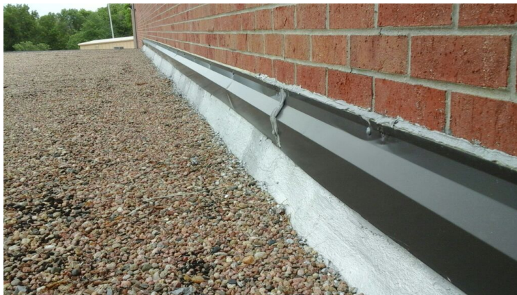
Photo showing condition of the perimeter flashings.
