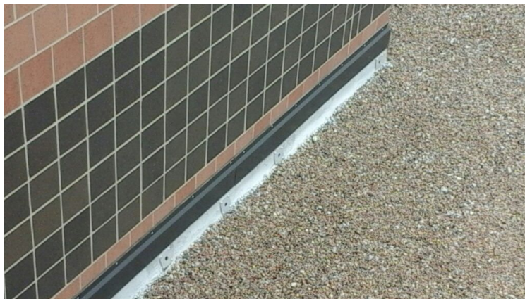
Photo showing condition of the perimeter flashings.
