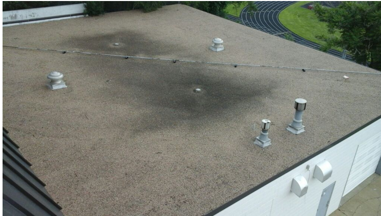
Photo showing overview of Area 03 Roof.
