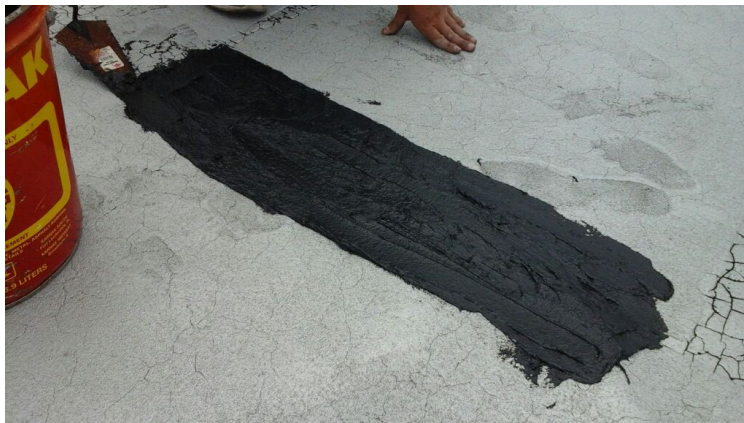
Photo showing repair made to the field.
