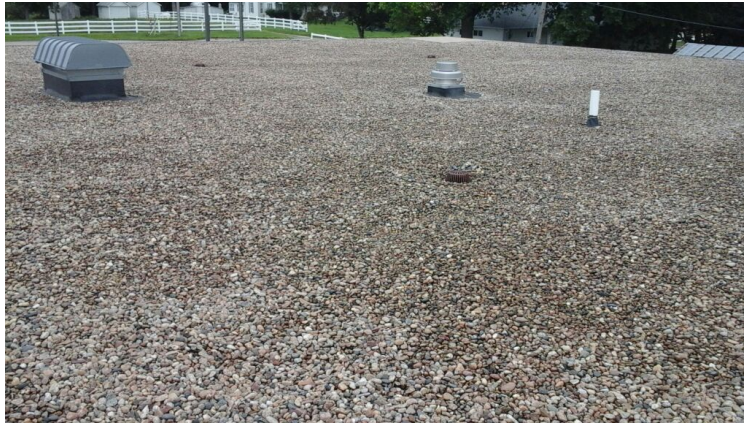
Photo showing overview of Area 03 Roof.
