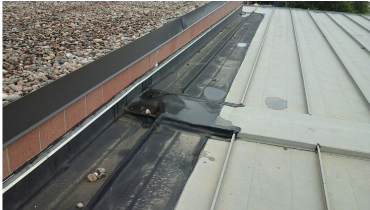
Photo showing perimeter with rubber between two roofs.
