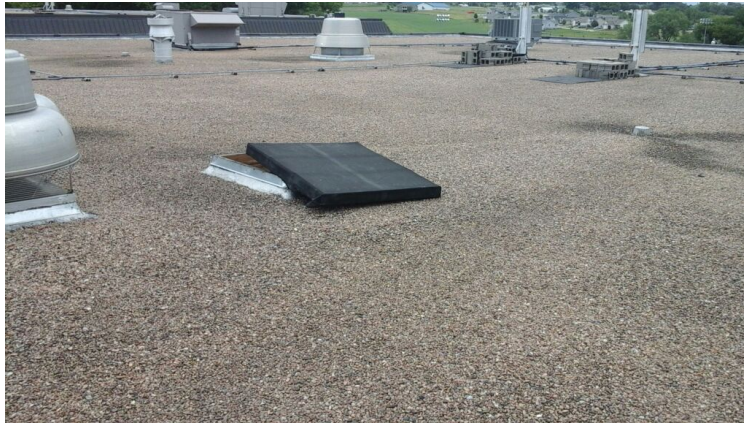
Photo showing overview of Area 04 Roof.
