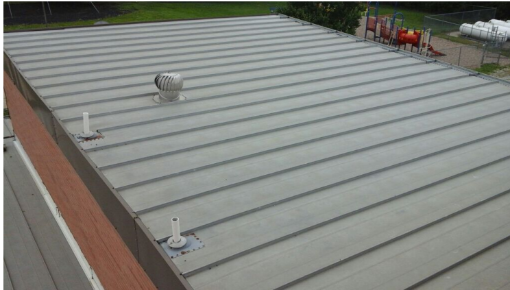
Photo showing overview of Area 11 Roof.
