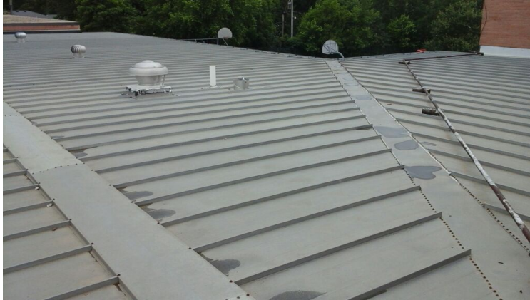
Photo showing additional overview of Area 02 Roof.
