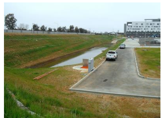
Example of Detention Area for Stormwater
