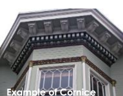
Example of Cornice
