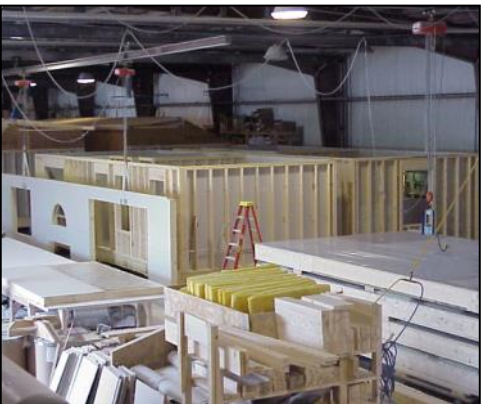
Example of a Dwelling, Manufactured Home Source: http://transportablehomesspecialist.com/
