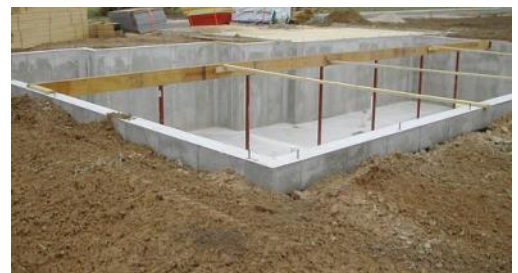
Example of a Permanent Foundation
