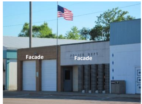
Example of a Facade
