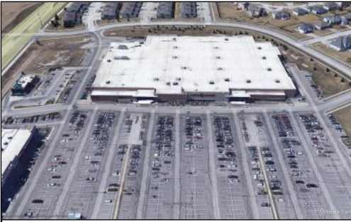
Example of Big Box Retail Store Source: Google Earth
