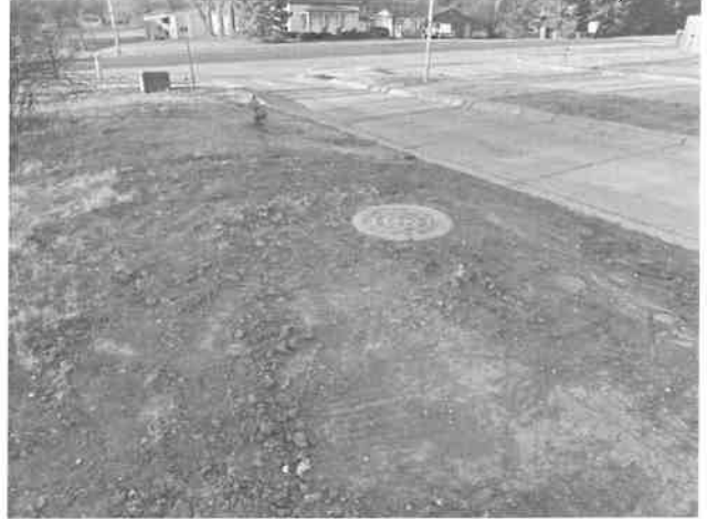
3/27: Manhole cover at Autumn Road.
