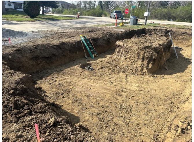
4/9: Booster pump station, foundation excavation.
