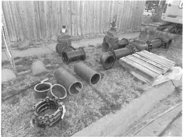
3/27: Piping for install at Autumn Parkway.
