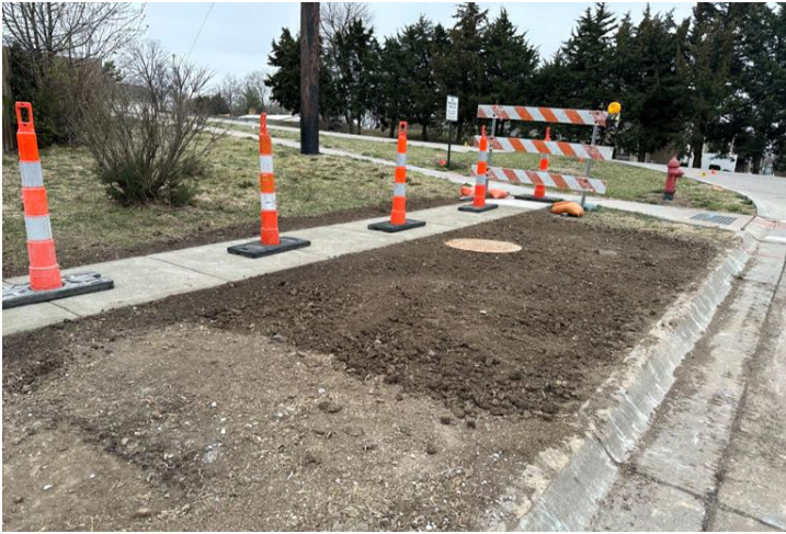
3/31: Backfill and sidewalk replacement on Autumn Parkway.
