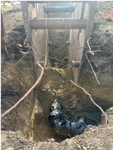
4/8: 12-inch suction line, photo looking east.
