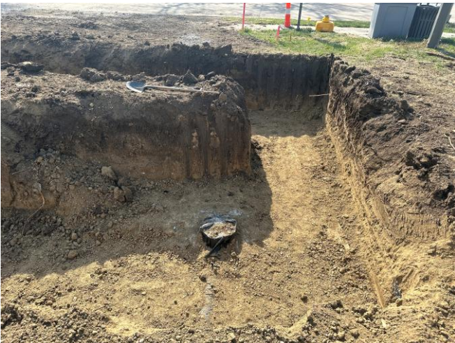
4/9: 12-inch discharge line connection at booster pump station.
