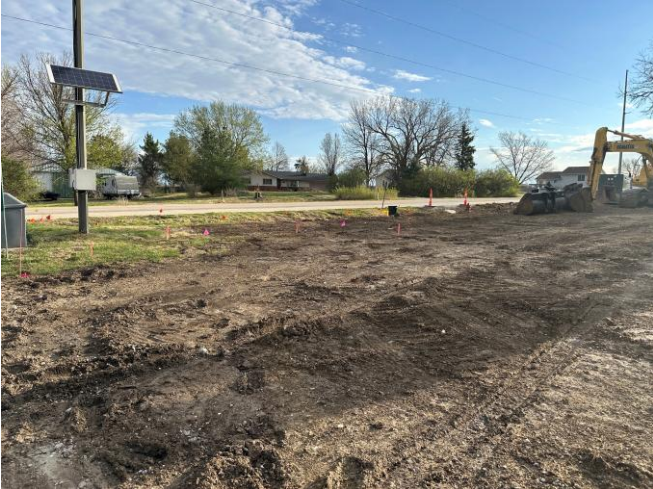
4/2: Construction staking of booster pump station.
