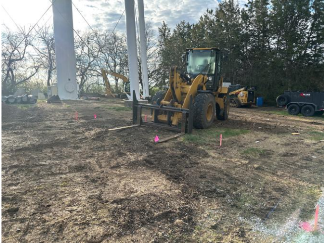
4/2: Construction staking of booster pump station.
