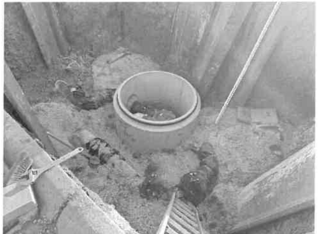
3/27: Check valve assembly and manhole installation at Autumn Parkway.
