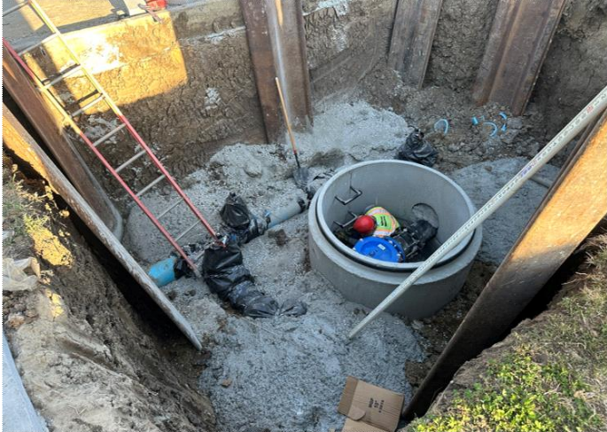
3/30: Continued installation of check valve assembly at Autumn Parkway.
