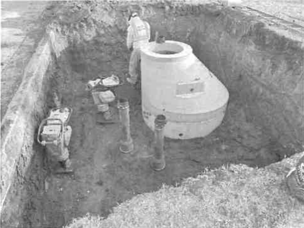
3/25: Backfill at check valve assembly on Autumn Road.
