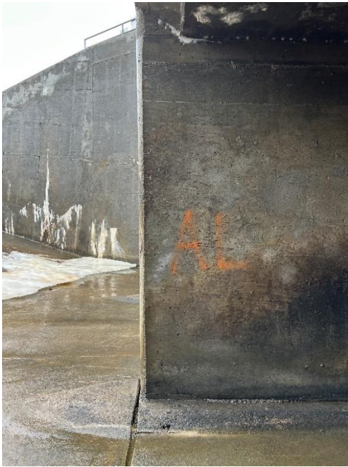
Location: Right Barrel – Joint A - Left Elevation
