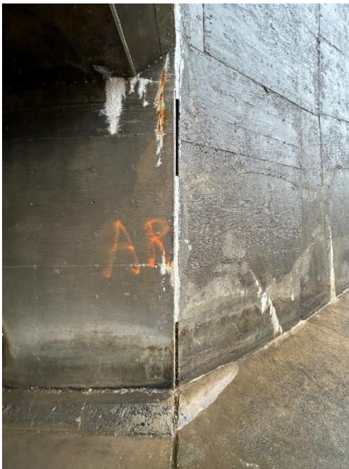
Location: Right Barrel – Joint A - Right Elevation
