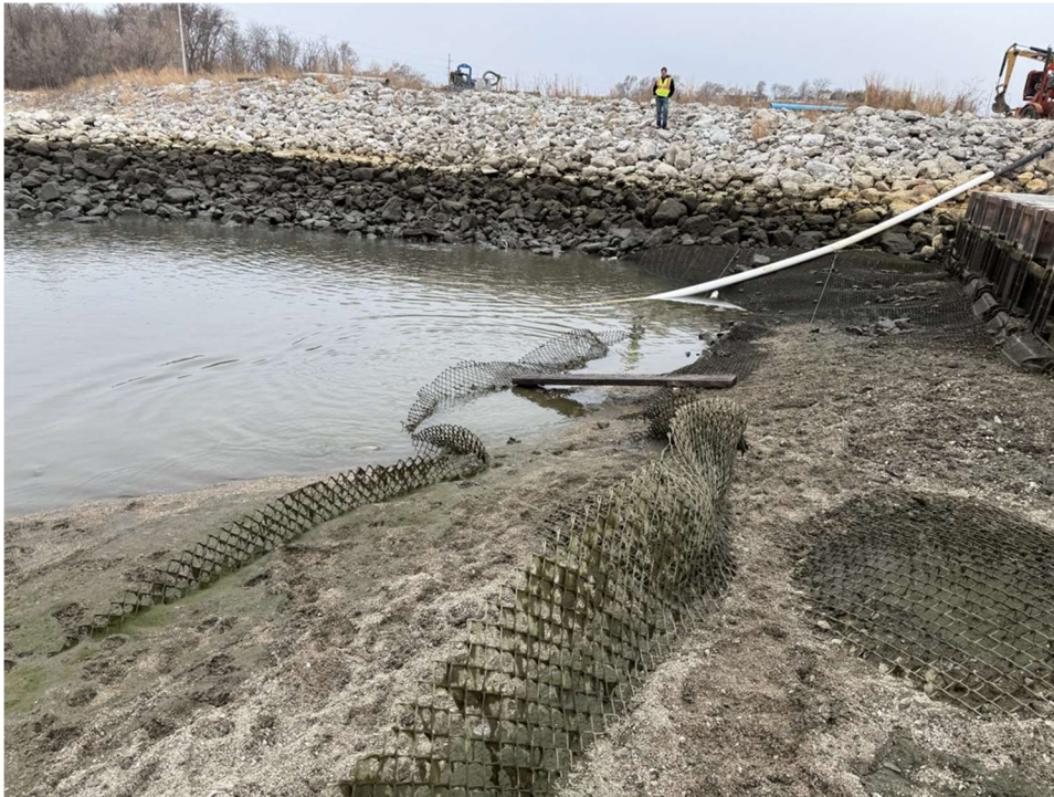
Stilling Basin Fencing
