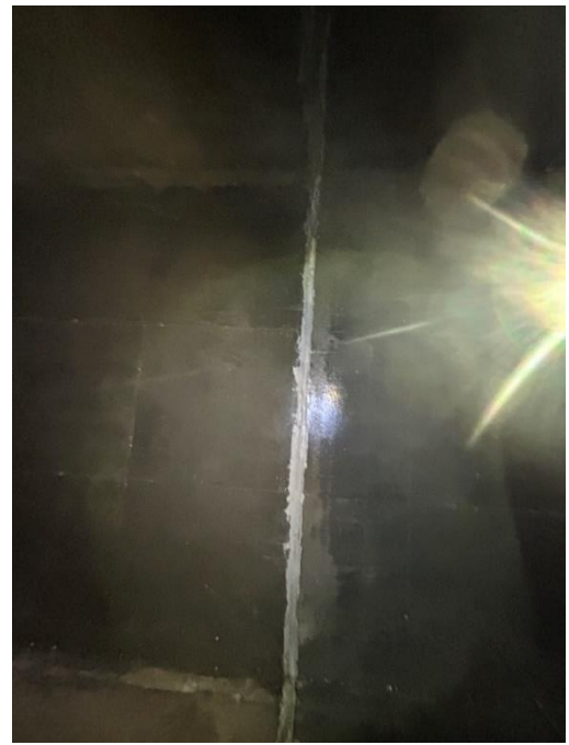
Location: Middle Barrel – Joint C - Top Elevation
