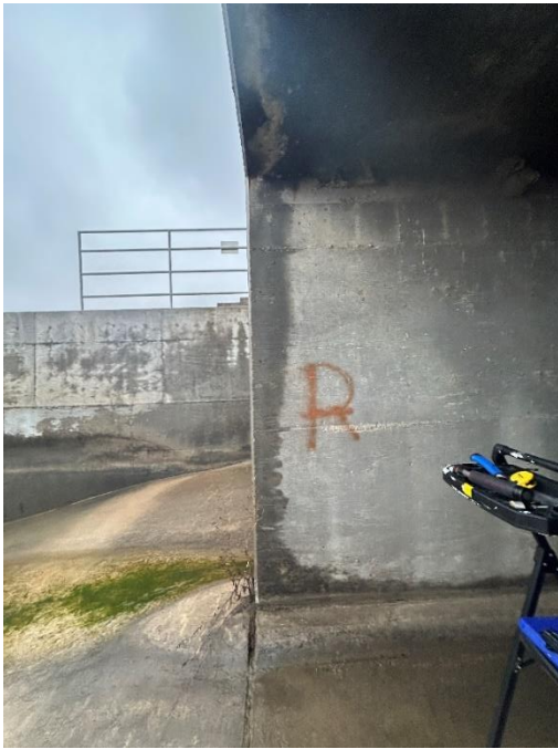
Location: Middle Barrel – Joint F - Right Elevation
