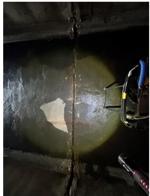
Location: Left Barrel – Joint D - Bottom Elevation Remarks: Joint filler in moderate condition. Joint Gap: 2.25” (typ.) with 3.5” gouge.
