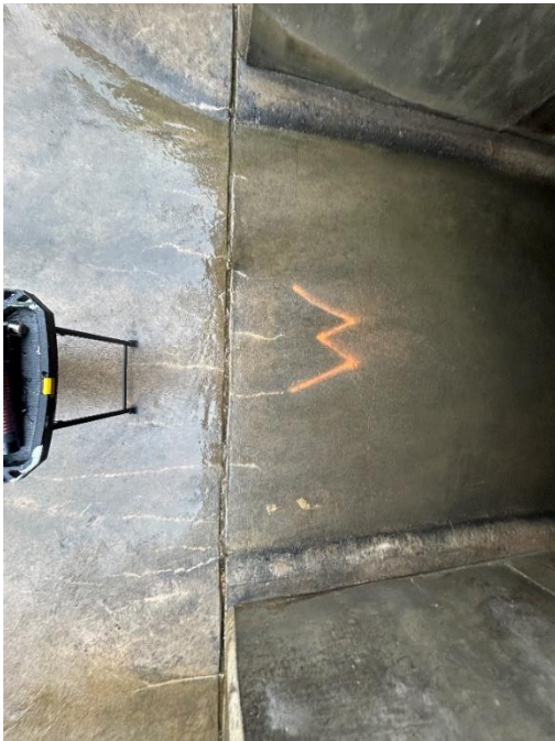
Location: Middle Barrel – Joint A - Right Elevation
