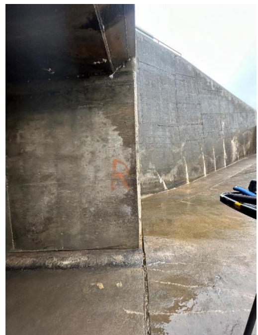
Location: Middle Barrel – Joint A - Bottom Elevation Joint Gap: 1.5" (typ.)
