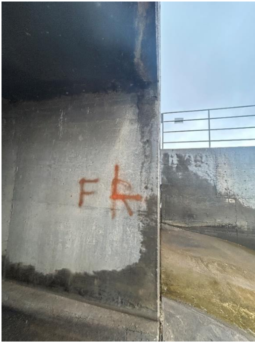
Location: Middle Barrel – Joint F - Left Elevation
