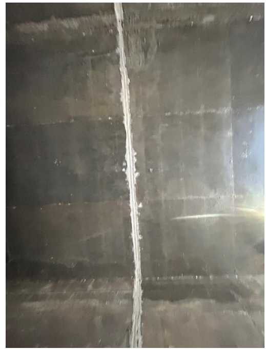
Location: Middle Barrel – Joint B - Top Elevation
