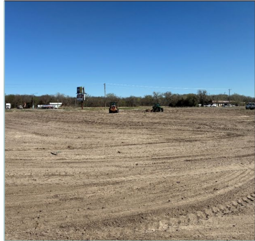
Current - Structures & debris have been removed.
