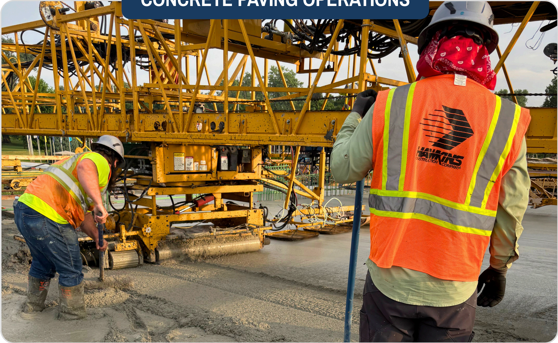
CONCRETE PAVING OPERATIONS
