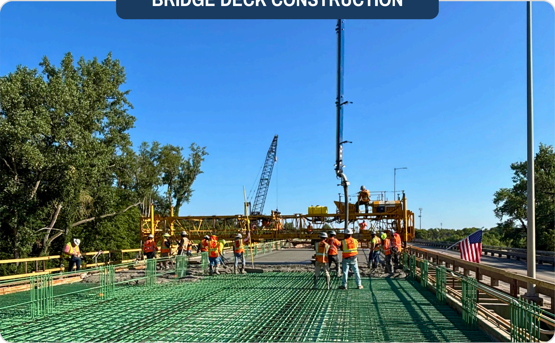
BRIDGE DECK CONSTRUCTION
