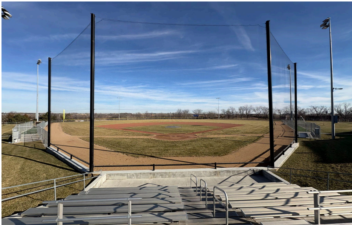
Picture Taken December 2025: The new grass infield is complete, but the grass has gone dormant.
