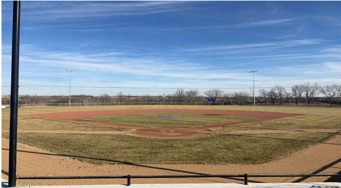
Picture Taken December 2025: The new grass infield is complete, but the grass has gone dormant.
