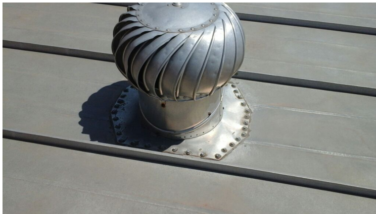
Photo showing condition of the projections.
