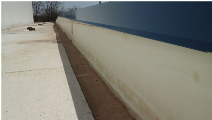
Photo showing condition of the perimeter flashings.
