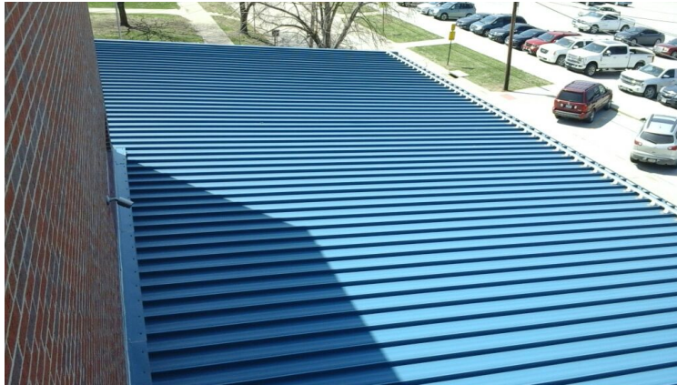
Photo showing overview of Area 04 Roof.
