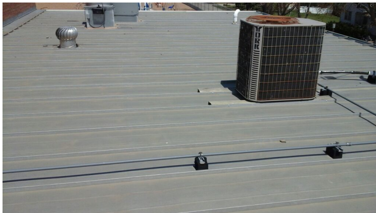
Photo showing additional overview of Area 10 Roof.
