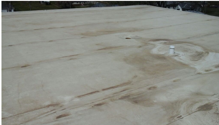
Photo showing additional overview of Area 05.
