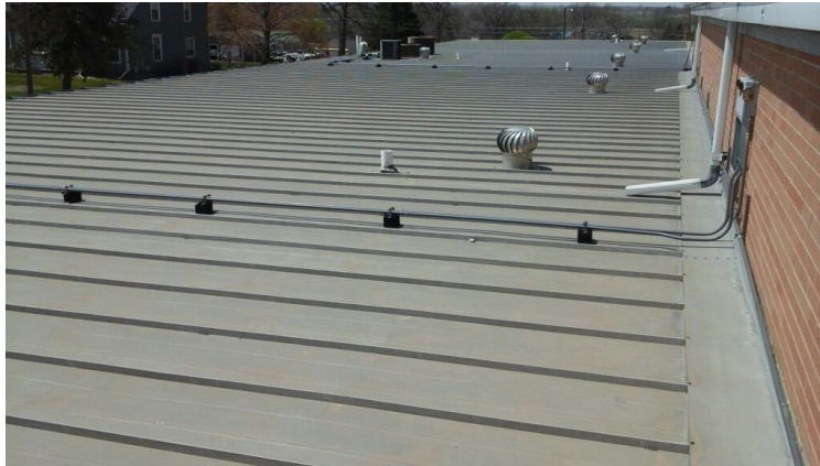
Photo showing overview of Area 10 Roof.
