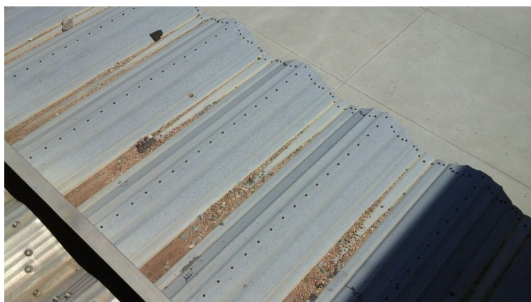
Photo showing overview of adjacent metal roof.
