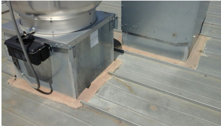
Photo showing projections with all soft sealant on flashing.
