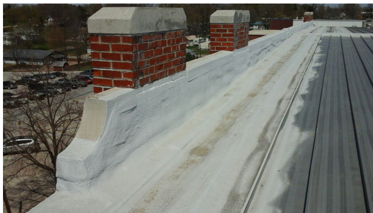
Photo showing spray foam along parapet wall.
