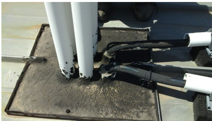
Photo showing a pitch pan that needs to be refilled and attended to.
