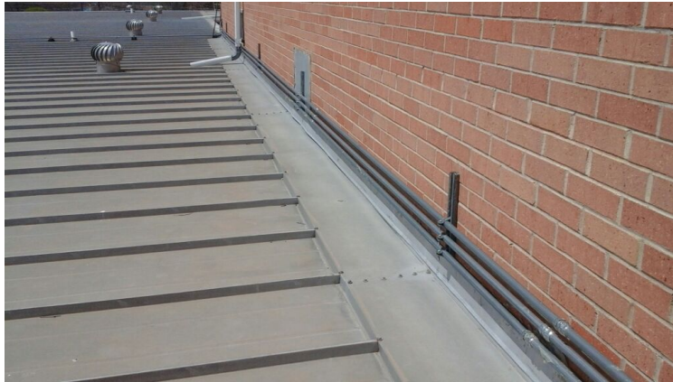
Photo showing condition of the perimeter metal.
