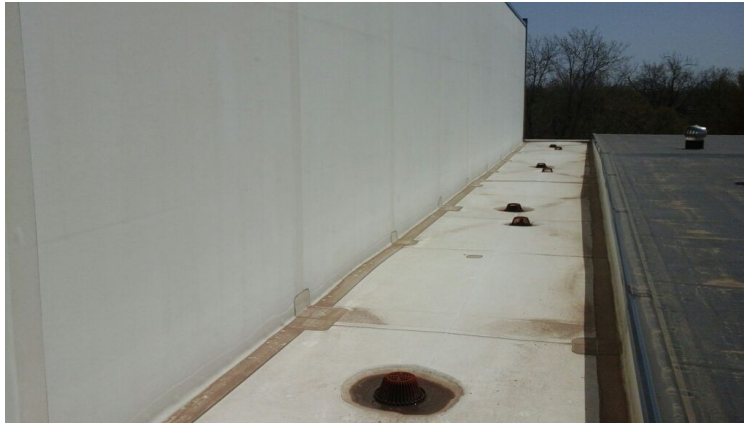
Photo showing overview of Area 03 Roof.
