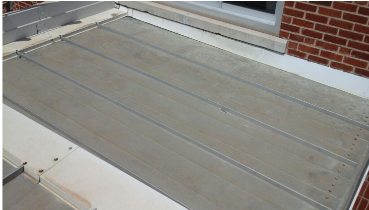
Photo showing overview of adjacent metal roof.
