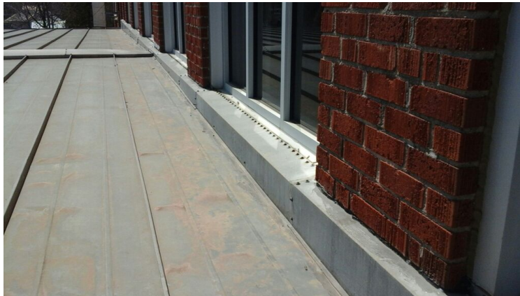
Photo showing condition of the perimeter metal.
