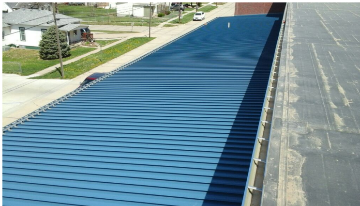
Photo showing additional overview of Area 04 Roof.
