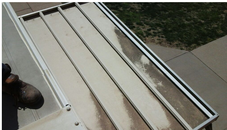
Photo showing overview of additional adjacent metal roof.
