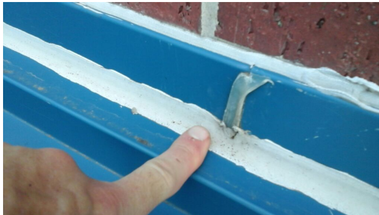
Photo showing caulking run right over old silicone seam.
