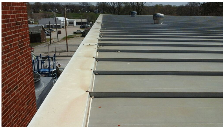
Photo showing condition of the perimeter metal.
