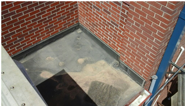
Photo showing additional overview of adjacent EPDM roof.
