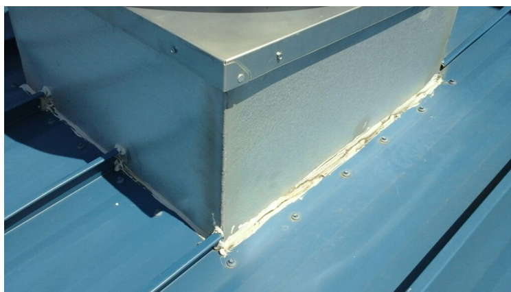
Photo showing condition of the projections.
