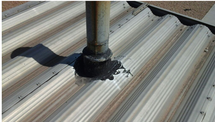
Photo showing vent stack covered in asphalt flashing.
