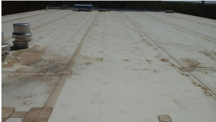
Photo showing overview of Area 01 Roof.
