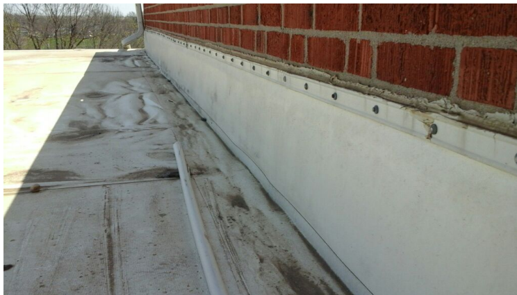
Photo showing condition of the perimeter flashings.
