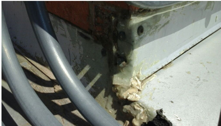
Photo showing repairs made with silicone to corner.
