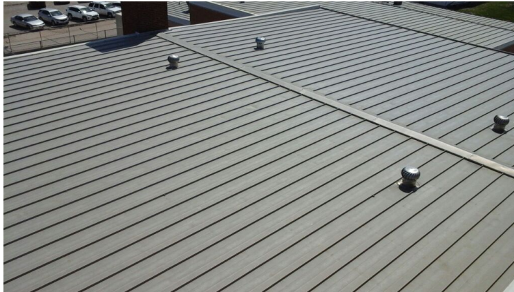
Photo showing overview of Area 08 Roof.
