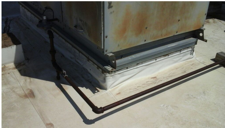
Photo showing condition of projection flashings.
