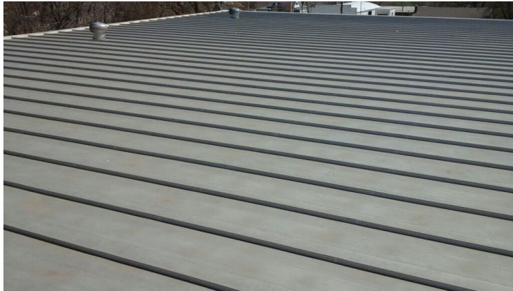
Photo showing overview of Area 10 Roof.
