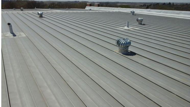
Photo showing overview of Area 06 Roof.
