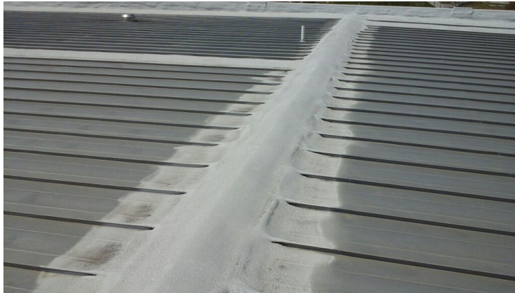
Photo showing spray foam along ridge cap.
