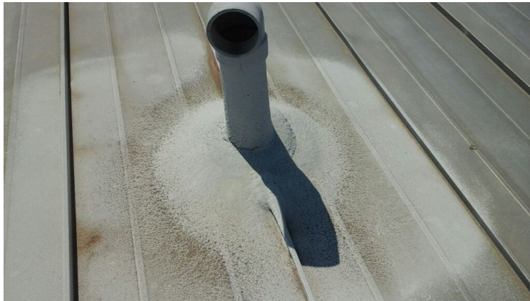
Photo showing spray foam on projection.
