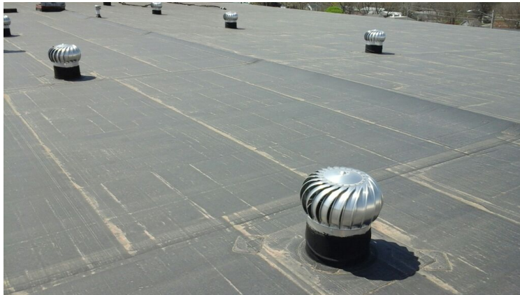
Photo showing condition of projection flashings.
