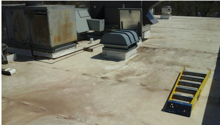
Photo showing overview of Area 05 Roof.
