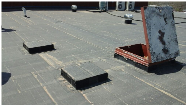
Photo showing condition of projection flashings.
