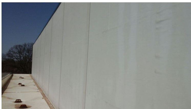
Photo showing condition of wall covered in EPDM.
