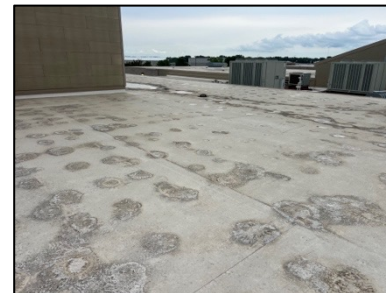
Rubber Membrane Roof
