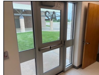
Interior Door View
