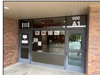
Eagle Main Entry Doors
