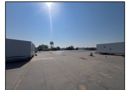
Rubber Membrane Roof
