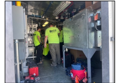
Heat Pump Installation 2025
