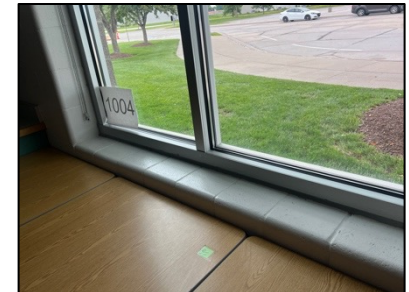
Interior Windows View
