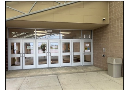
High School Entry Doors
