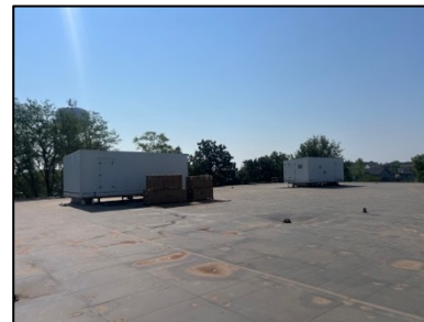
Rubber Membrane Roof
