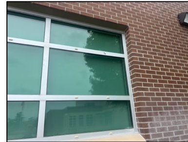
Typical Aluminum Window Frame
