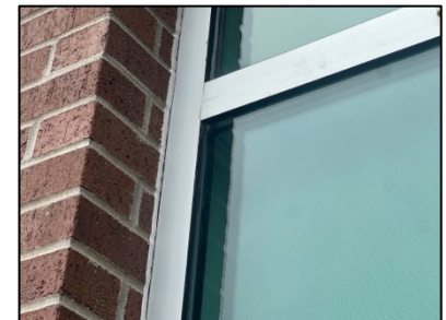
Caulked 2007 Aluminum Windows
