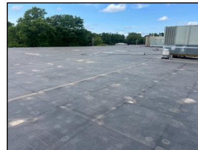
Rubber Membrane Roof
