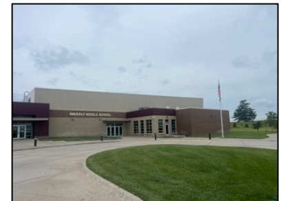
Full View West Middle School Entry
