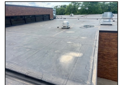
Rubber Membrane Roof
