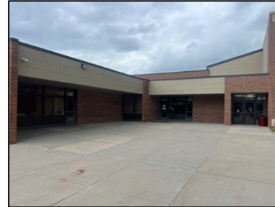
Eagle Main Entry
