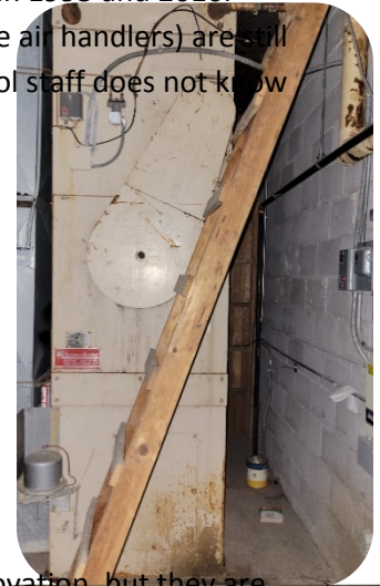
Old Gym AHU (One of Two) – Original to 1967 construction, and no longer in service.
