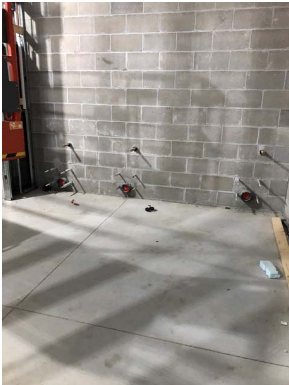
Toilet rough-in Girl's Locker Room
