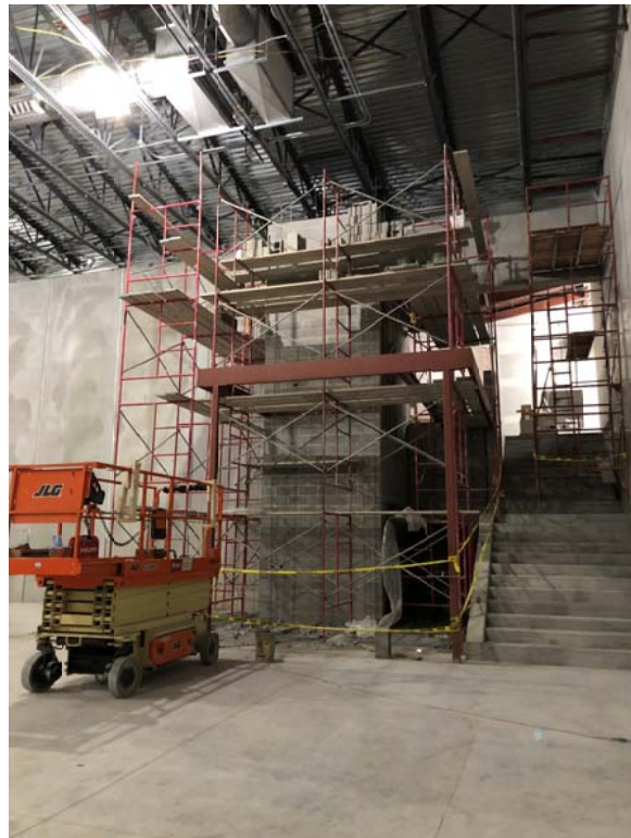
Elevator Shaft progress
