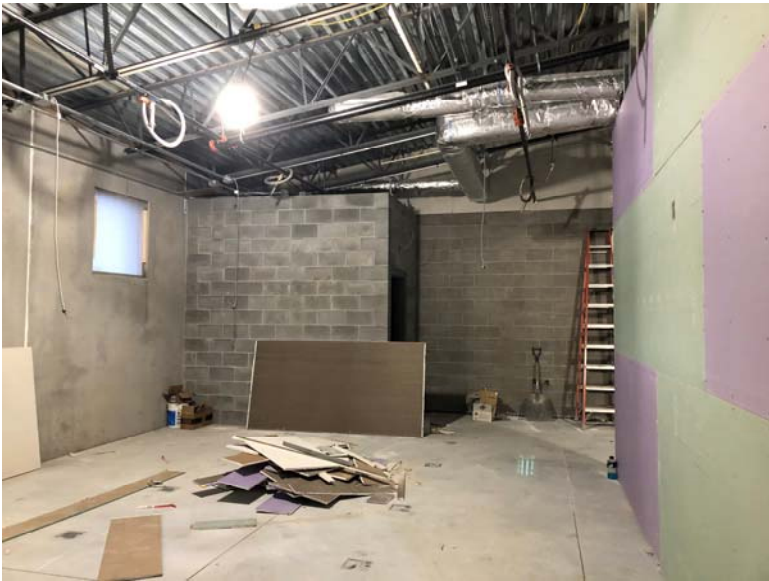
Girl's locker room seating area looking north
