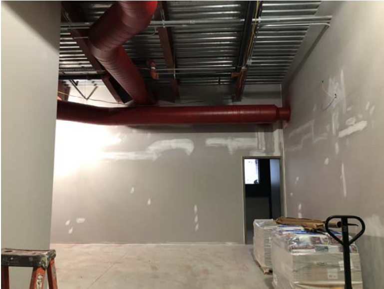
Concessions and restrooms area looking west
