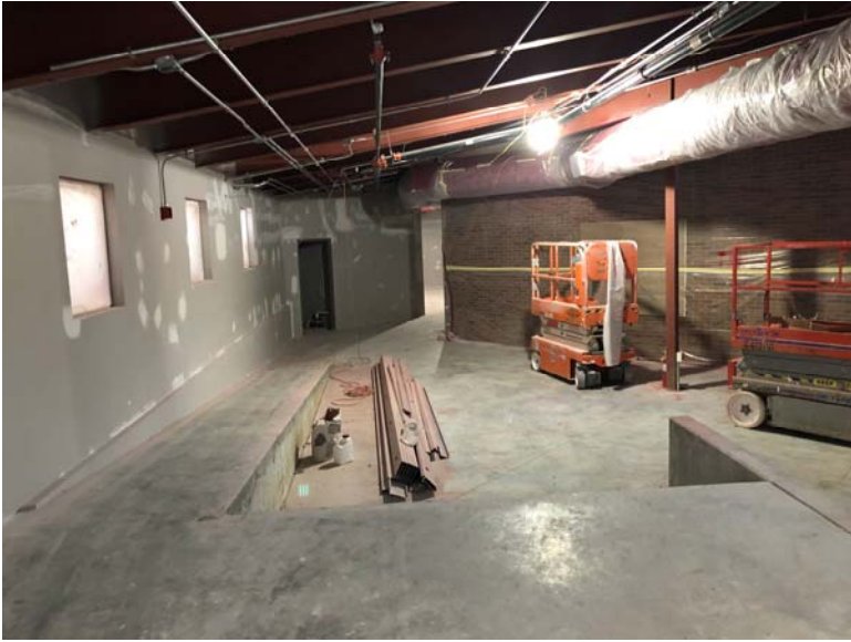
Entry tower stairs and ramp
