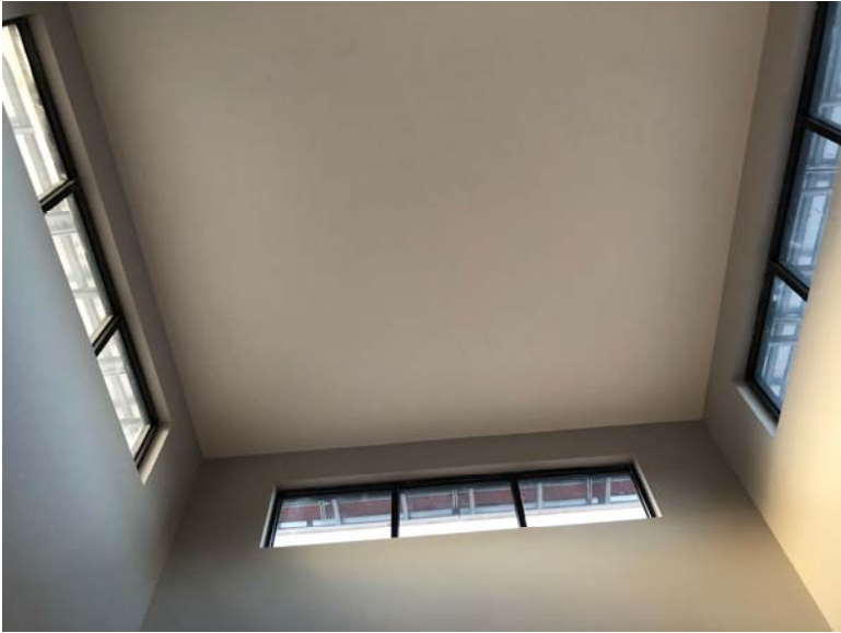
Entry tower clerestory windows
