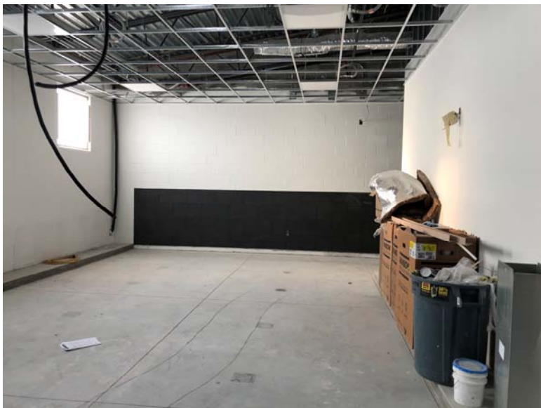
Gym looking east
