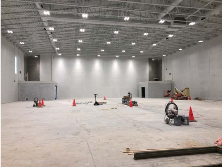
Gym looking east
