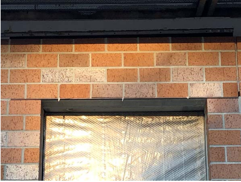
Window flashing, lintel, and weep detail
