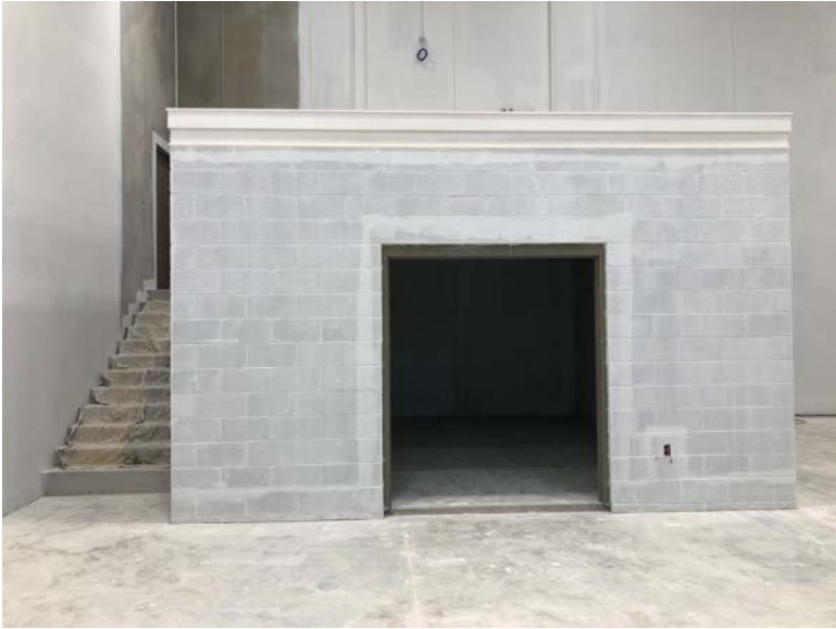
Gym small storage area
