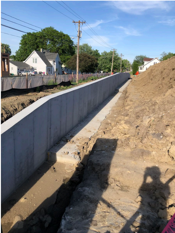
Retaining wall North of parking lot
