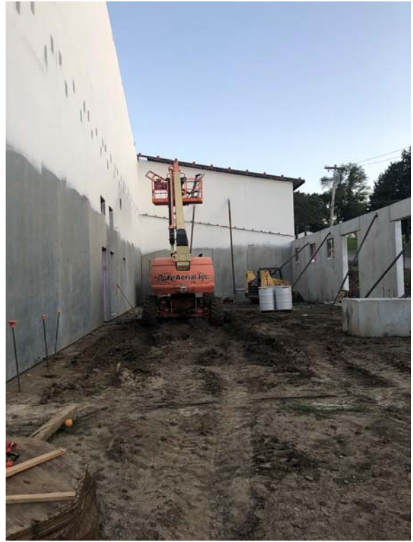
Locker Room area looking South. Weather barrier being applied.
