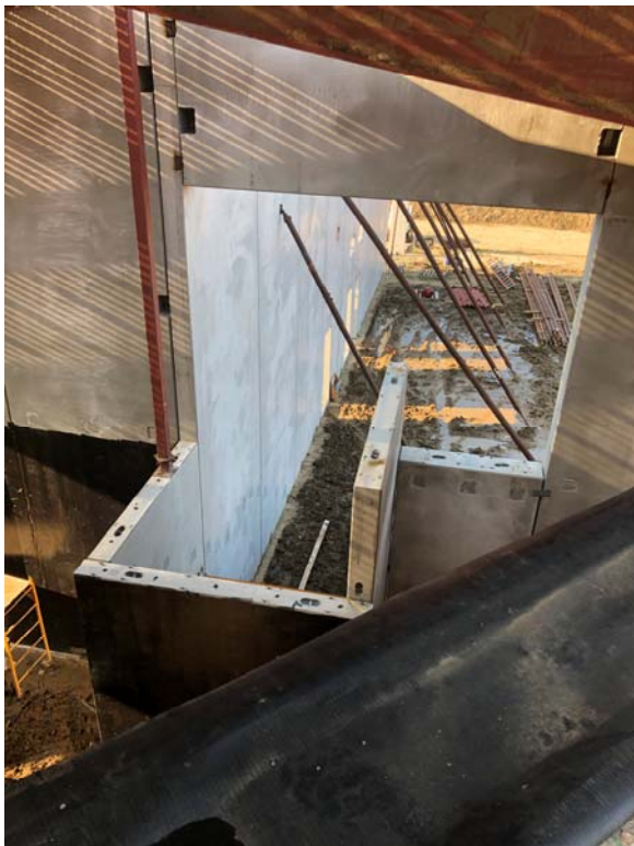
Commons to Gym stair location. Below grade Water proofing being applied.
