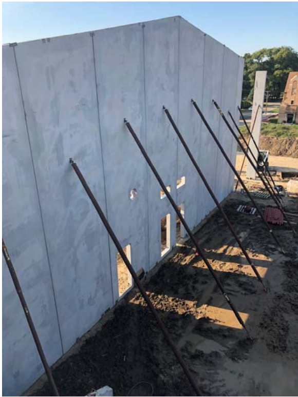
Gym West pre-cast concrete wall
