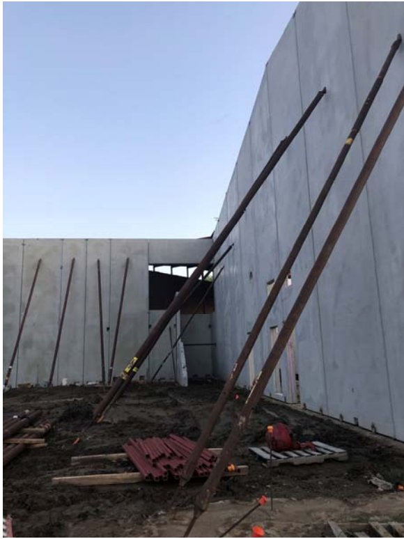
Gym West & South wall looking South
