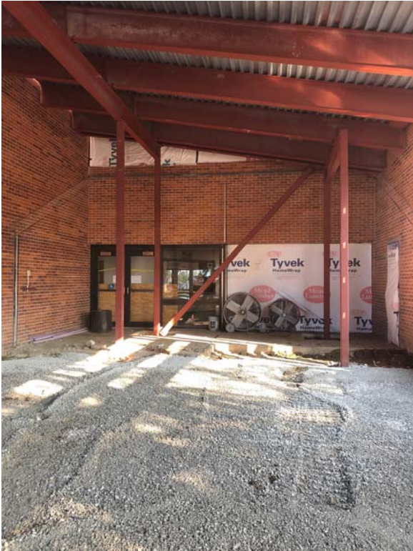
Commons interior looking South
