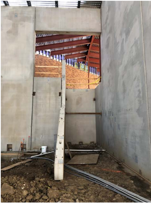
Gym to Commons stair location
