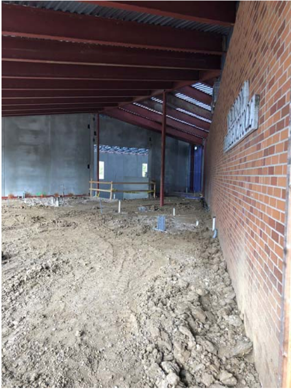
Concessions under slab plumbing
