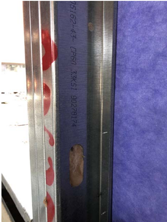
Pre-insulating concealed spaces
