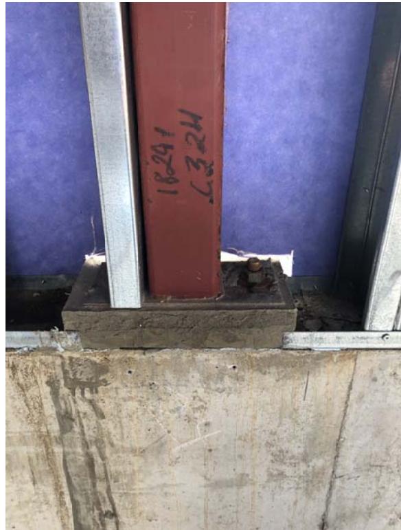
Grout at column
