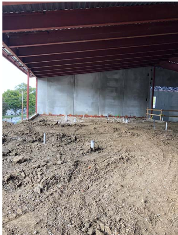
Restroom under slab plumbing
