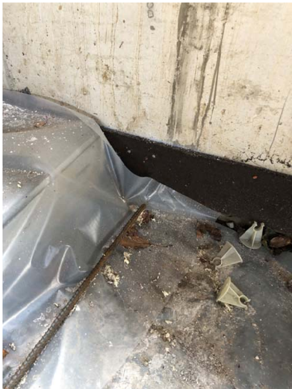
Expansion joint at slab abutting wall
