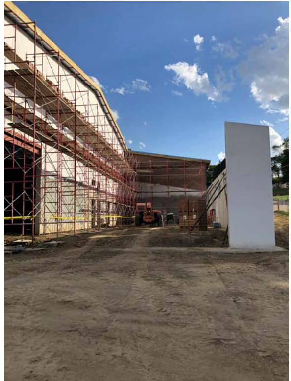
Locker room area
