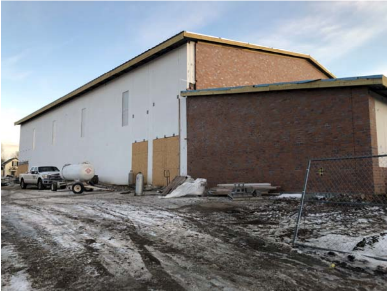
Gym & Locker Rooms looking southeast
