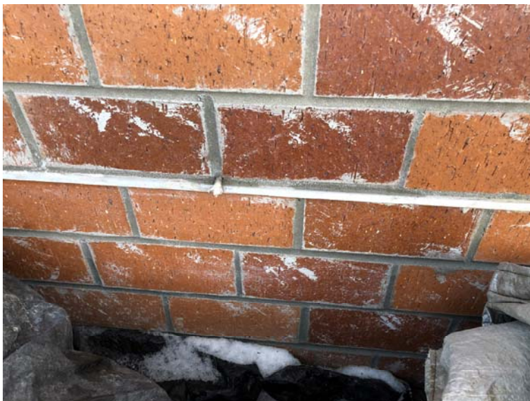
Base flashing and weeps
