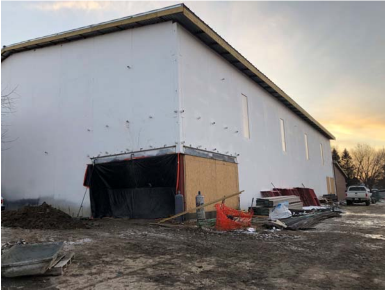
Gymnasium main entrance
