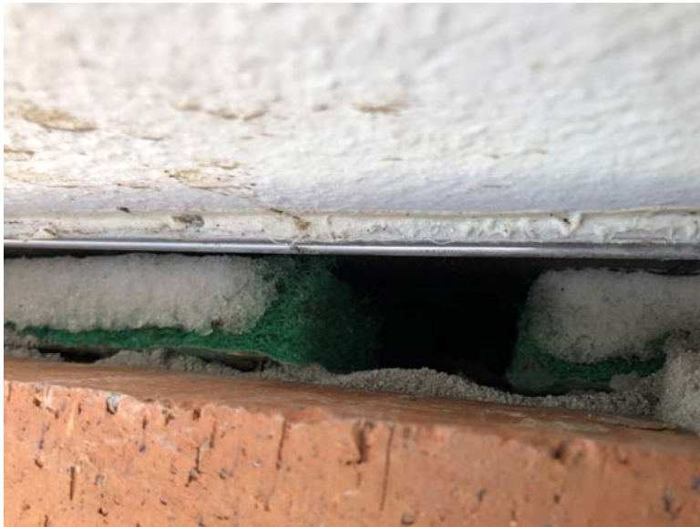
Mortar net & base flashing
