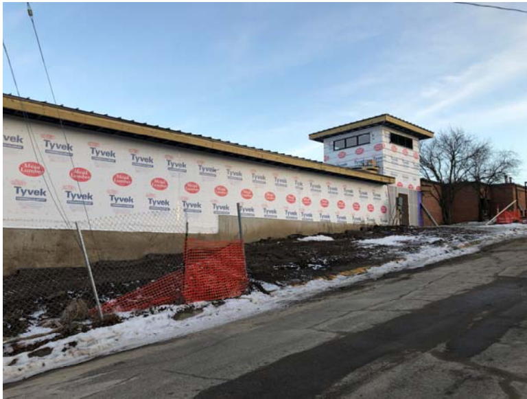
Restrooms and Concession area looking southeast
