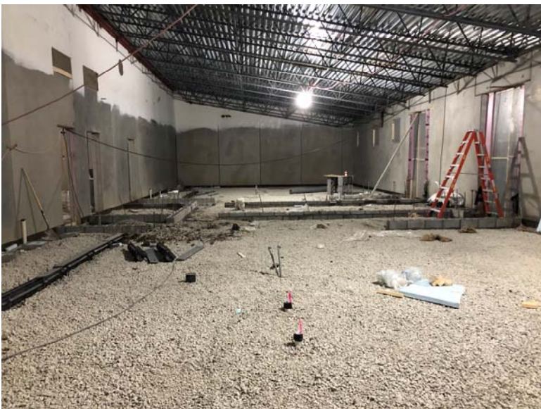
Locker rooms interior
