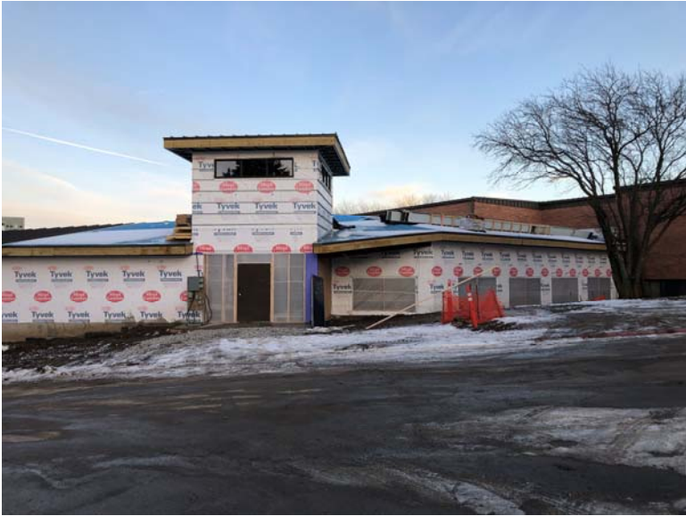
Commons exterior looking east
