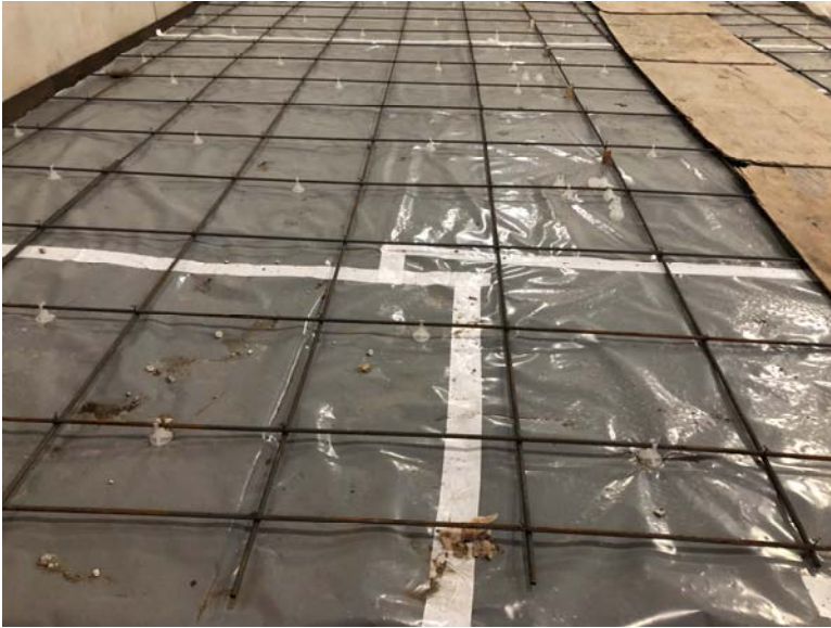
Gymnasium floor prep vapor barrier sealed, reinforcing properly chaired
