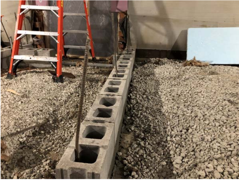
Reinforcing in CMU walls
