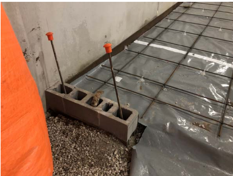
Expansion joint at slab perimeter
