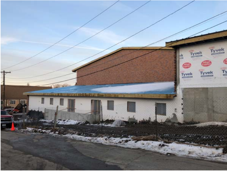
Locker Rooms looking northeast
