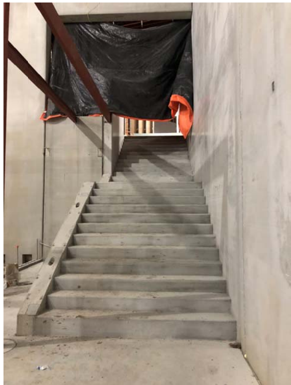
Stair to Mezzanine
