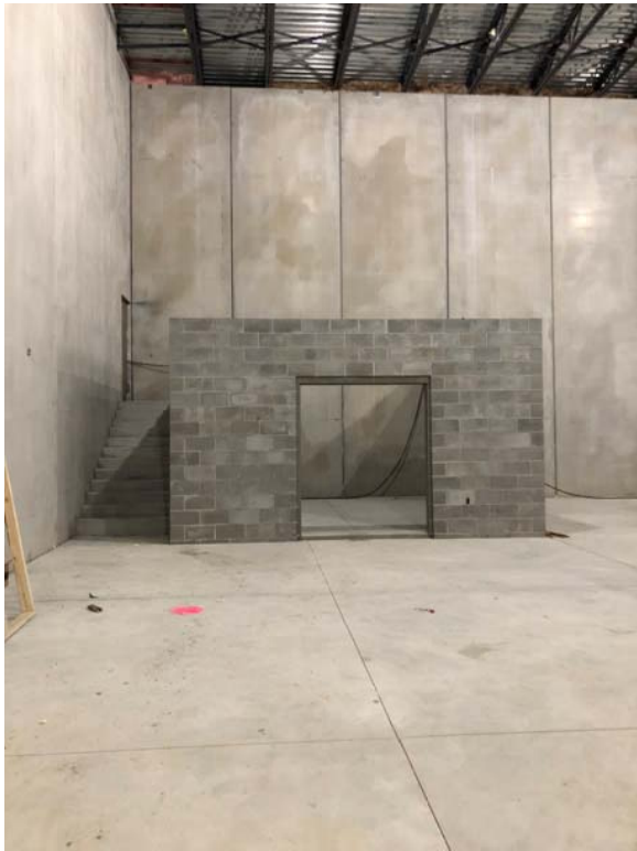
Gym SE storage room
