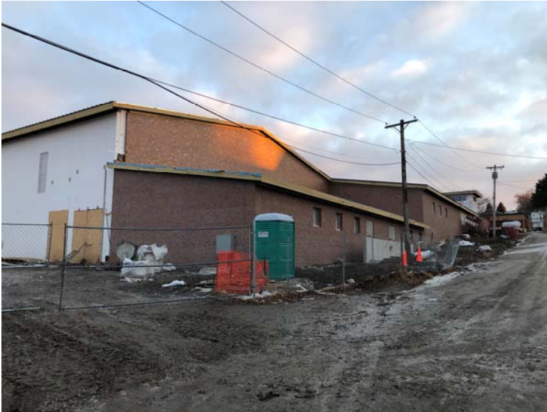
NW corner looking SE
