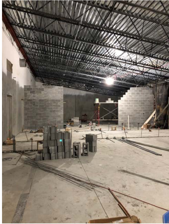
Locker room looking south
