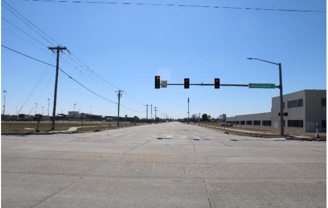
STUBBEMAN AVENUE LOOKING SOUTH FROM ROCK CREEK RD. (SUBJECT SITE TO LEFT IN FOREGROUND)
