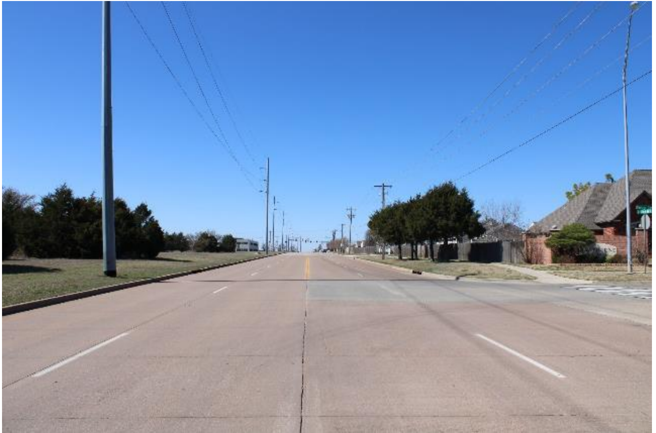
ROCK CREEK ROAD LOOKING WEST FROM HAMDEN AVENUE (SUBJECT SITE TO LEFT IN FOREGROUND)
