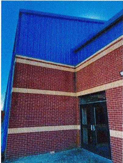
Water appears to have infiltrated the wall and is running from beneath the Z flashing and wall panel
