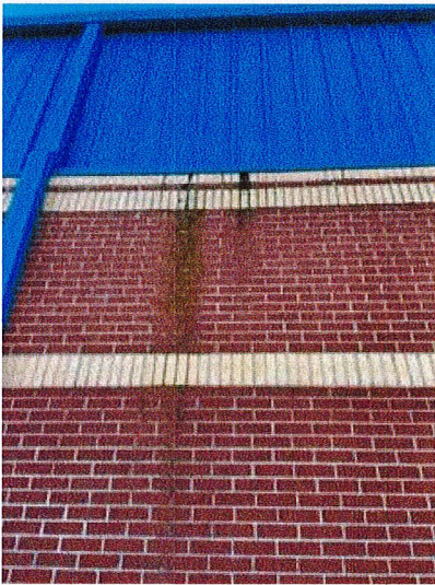
Water appears to have infiltrated the wall and is running from beneath the Z flashing and wall panel
