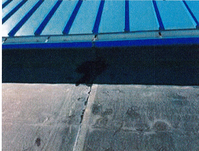
EPDM Rubber Membrane Flashing appears to be shrinking due to UV Light exposure
