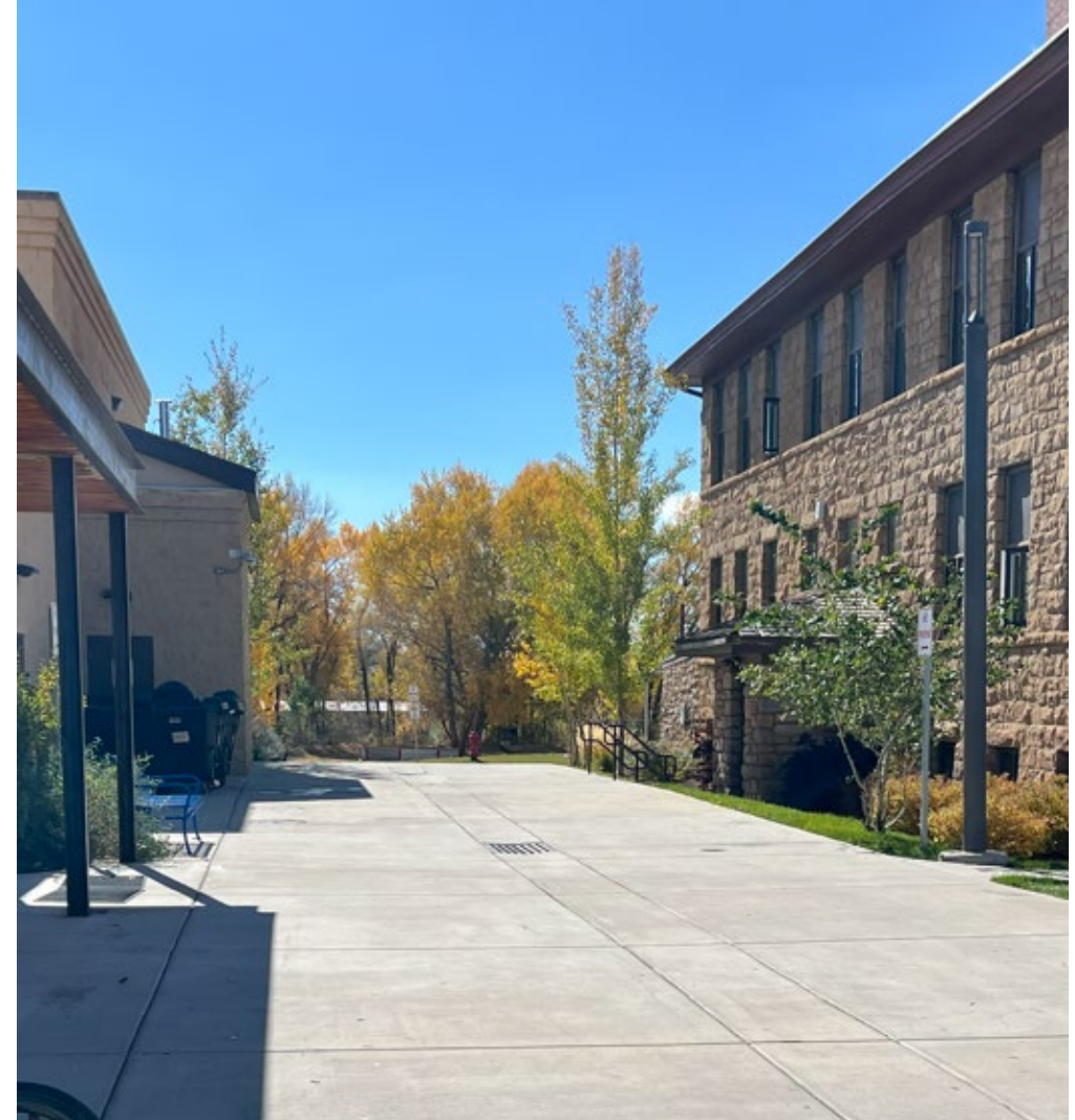
Perimeter area east of HS is unsecured
