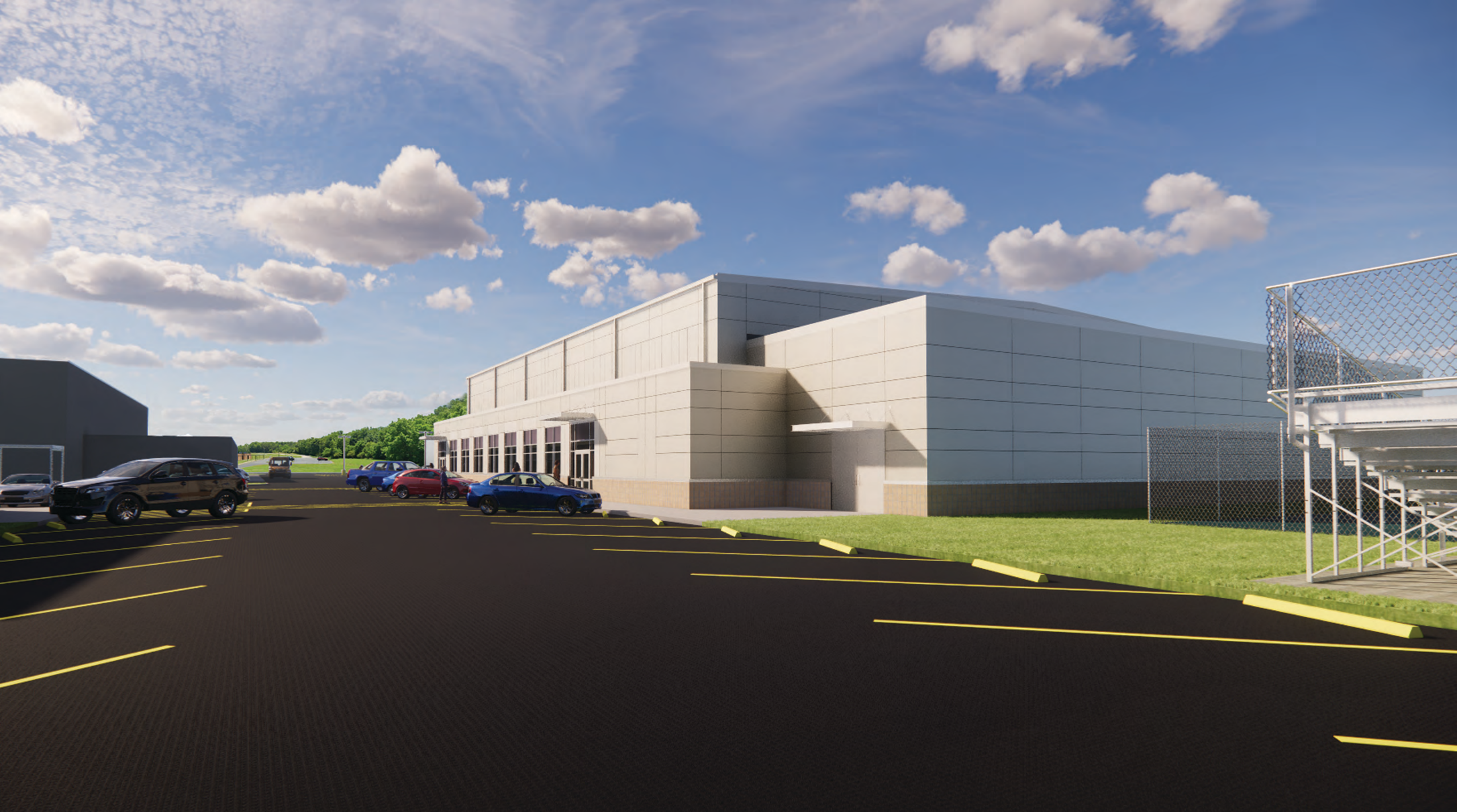
NEW AUDITORIUM FOR CUMBERLAND COUNTY HIGH SCHOOL REAR OF BUILDING
