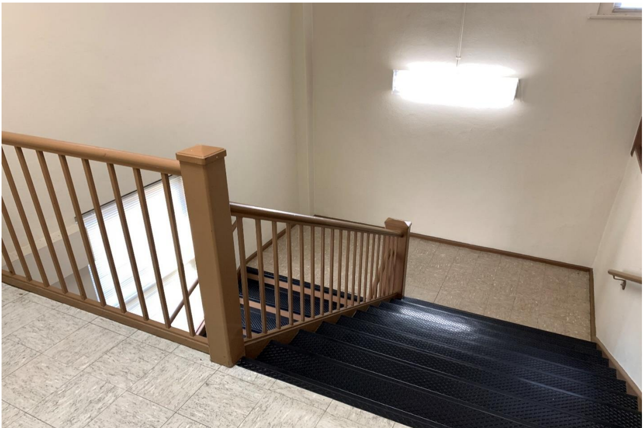
Building Stairwell (4 Levels)
