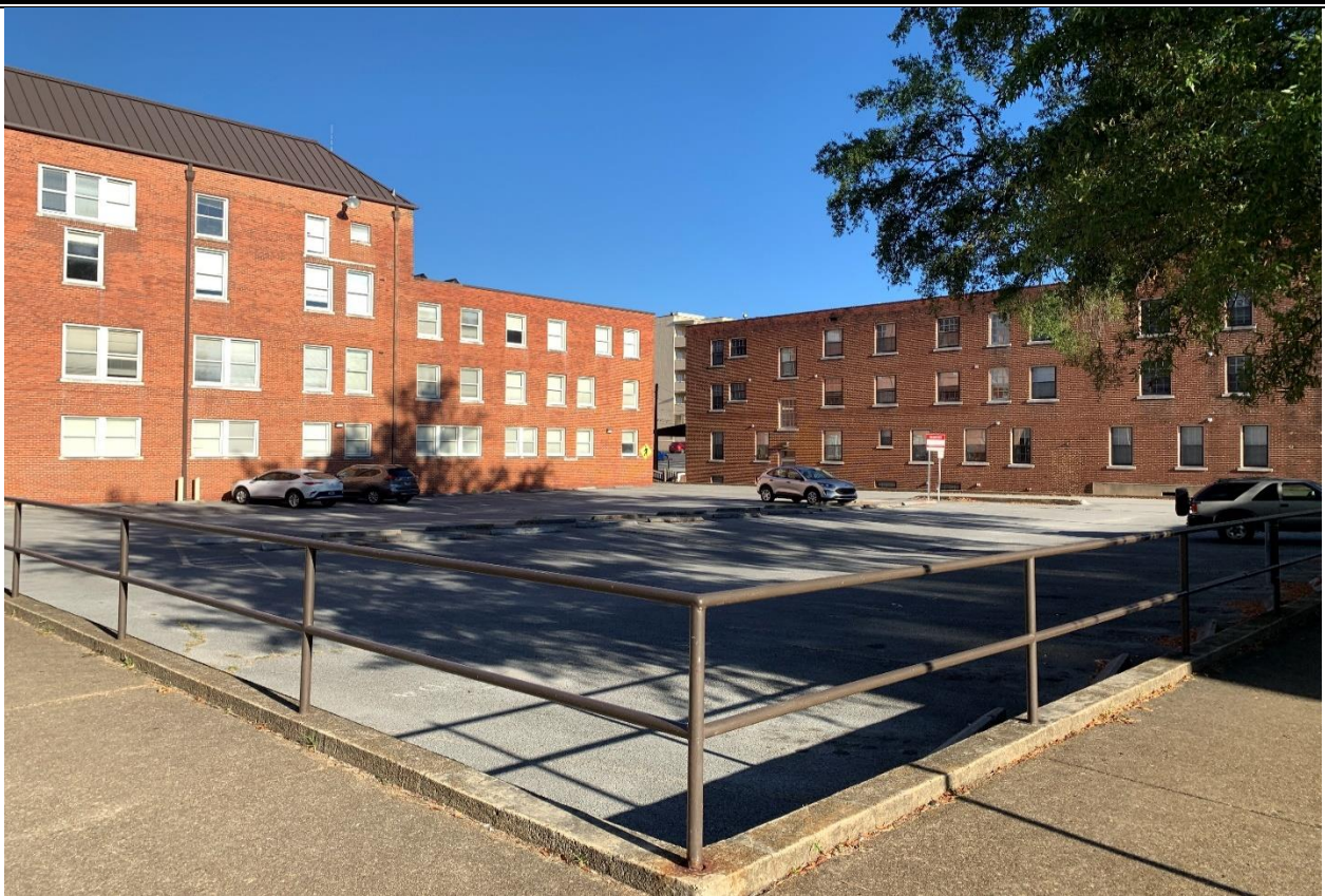
Subject Surface Parking Lot
