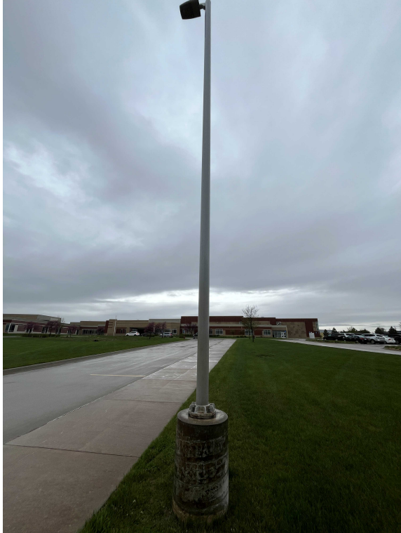
Intact light pole and concrete pier
