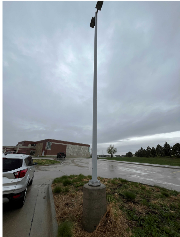
Intact light pole and concrete pier
