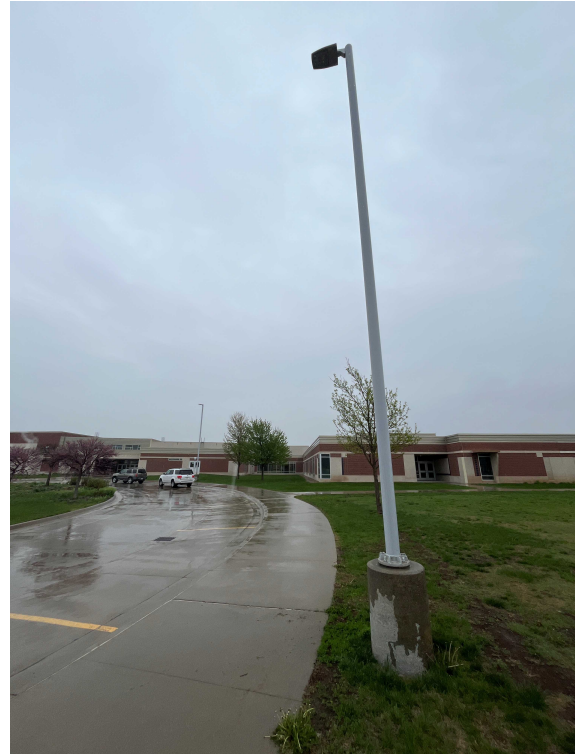
Intact light pole and concrete pier
