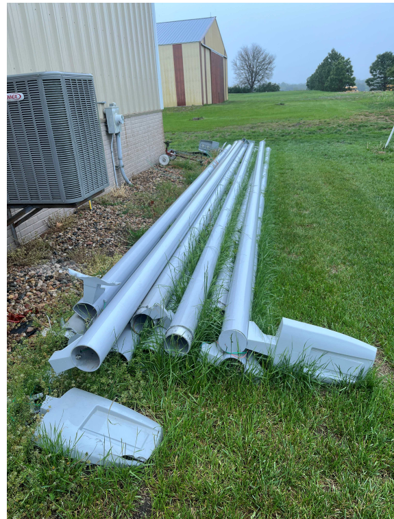
Failed light poles
