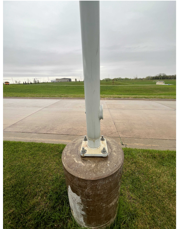
Reinstalled light pole with new base plate
