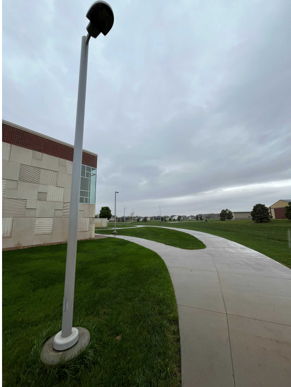
Intact light pole and concrete pier
