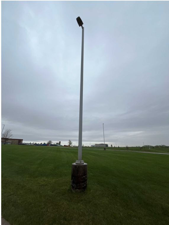
Intact light pole and concrete pier
