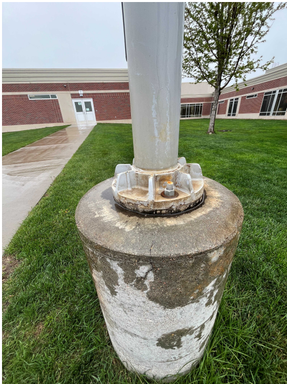
Intact light pole and concrete pier
