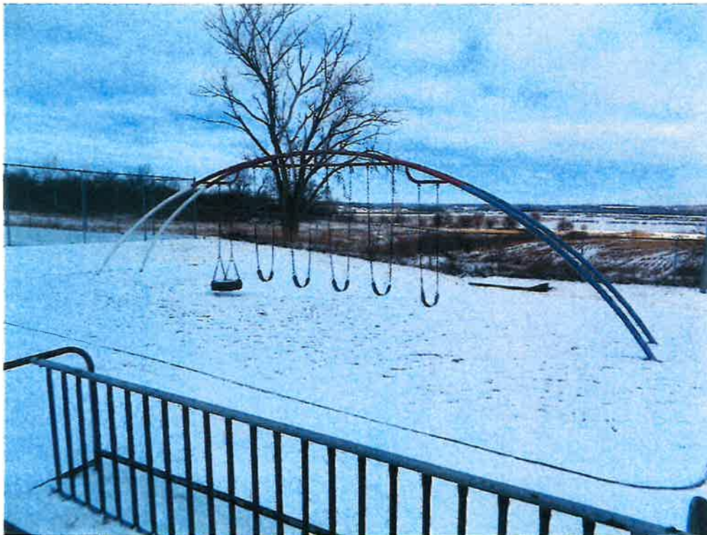
Tire swings are only allowed on a frame by itself. Very specific safety standards have to be followed on this type of swing.
