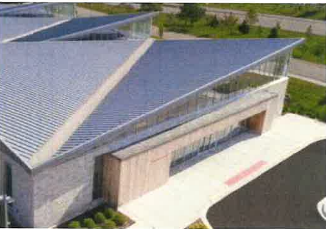
STANDING SEAM METAL ROOF
