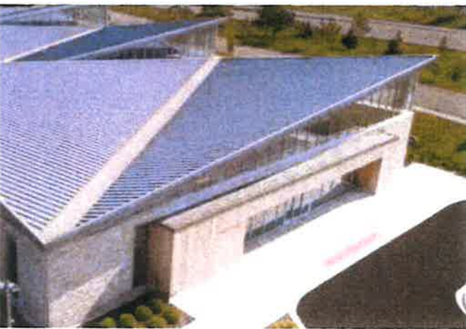
STANDING SEAM METAL ROOF
