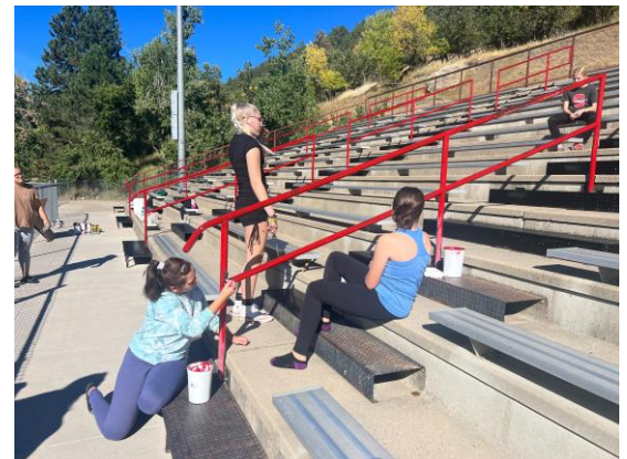
Painting the railings at Woodle Field.
