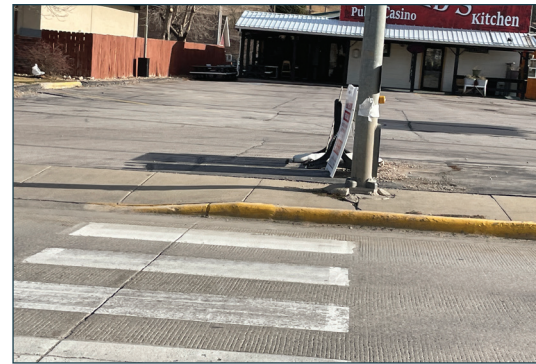
Crosswalk present, no ramp
