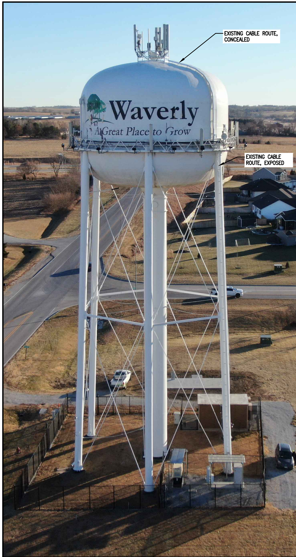
1 OVERALL TOWER PHOTO
