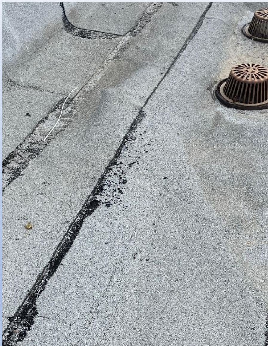
Image 3. Evidence of bubbling.
