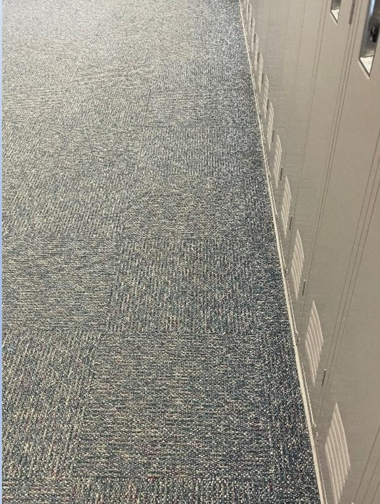
Image 1. Wear and discoloration. You can see the original color on the far right by the locker base.
