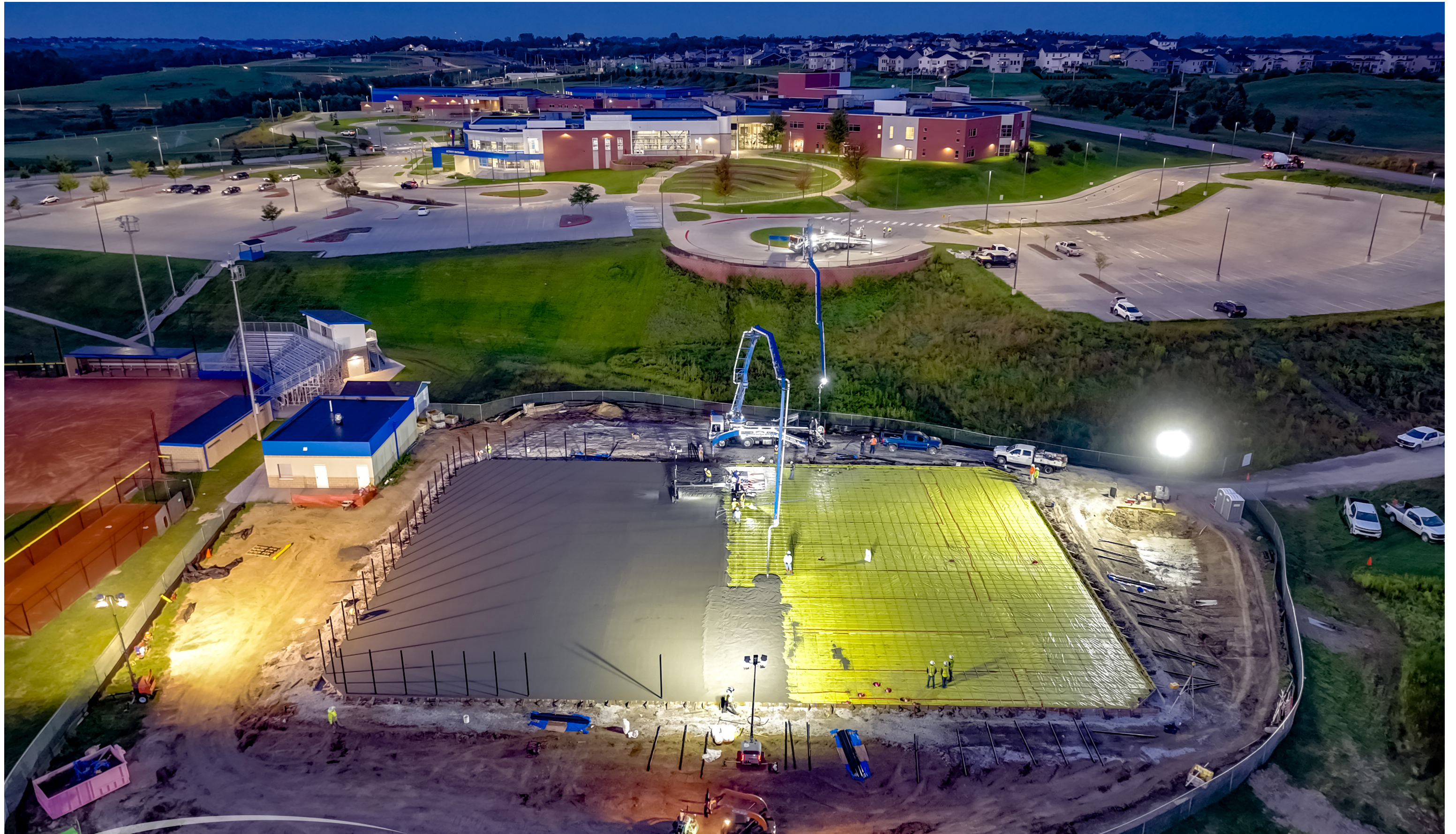
Bennington High School #2 | Tennis Court Progress 08 September 2025
