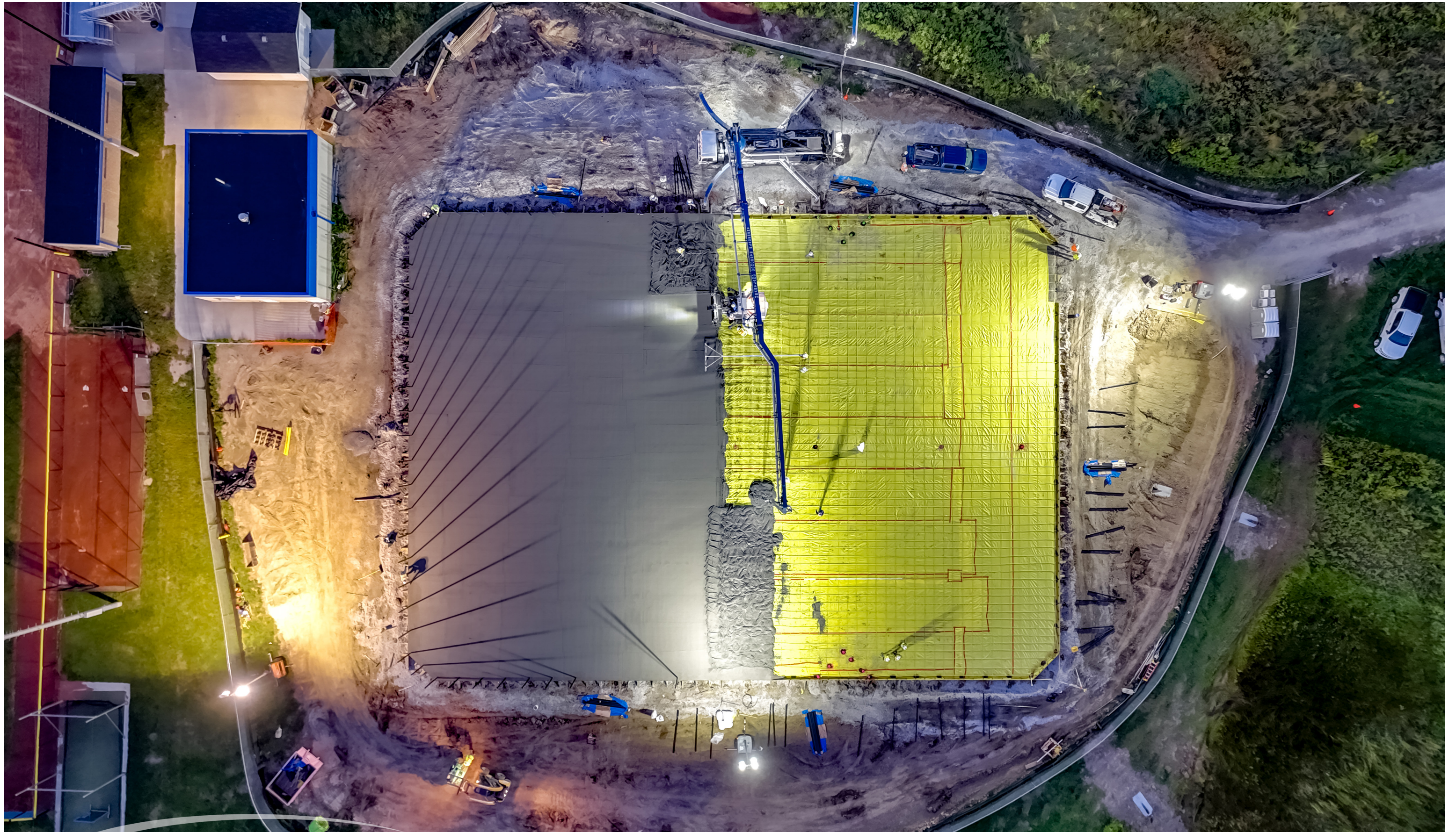
Bennington High School #2 | Tennis Court Progress 08 September 2025
