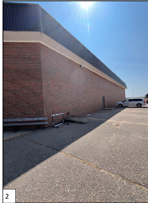
Building Exterior Looking Northeast
