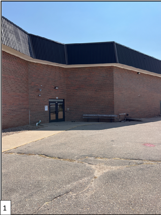
Exterior of Stair Wall
