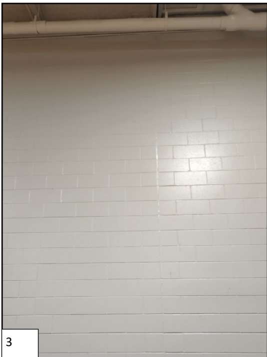
Interior of Gym Wall (Showing Control Joint)
