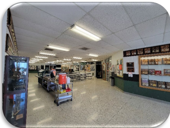
Typical Grid-Mounted Light Fixtures
