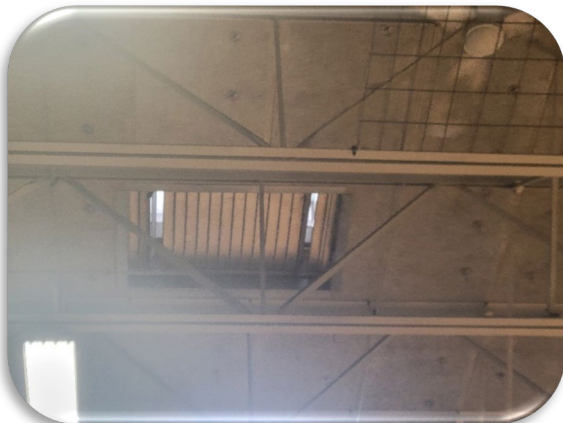
Gym Relief Damper – Blades stick open, rattle in the wind, etc
