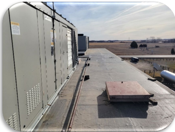
Install Safety Rail for Gymnasium Roof Hatch & Equipment
