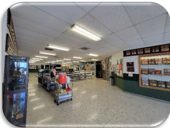
Typical Grid-Mounted Light Fixtures
