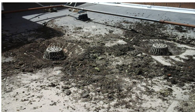
Cleared out drains.
