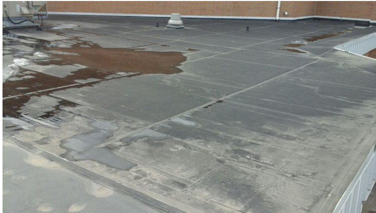
Photo showing overview of Area 13 Roof.
