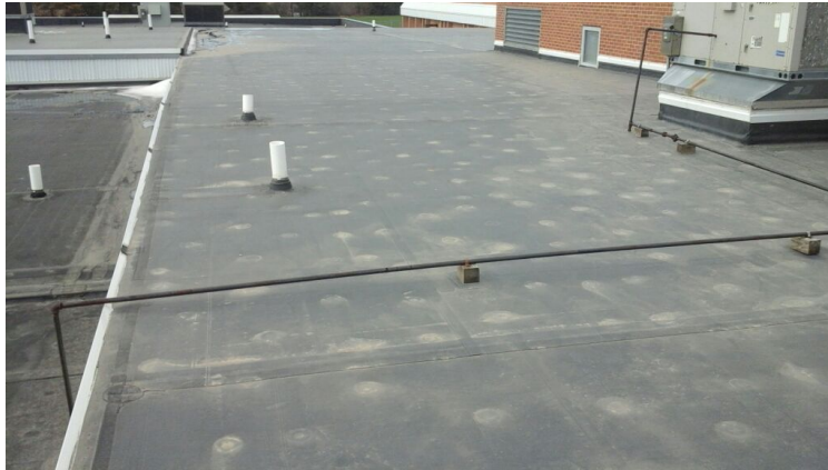
Photo showing overview of Area 04 Roof.
