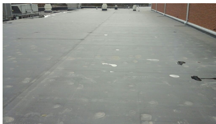
Photo showing an additional overview of Area 04 Roof.
