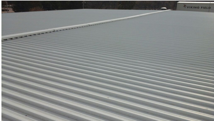
Photo showing overview of Area 08.
