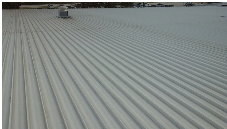
Photo showing an additional overview of Area 09 Roof.
