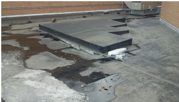
Photo showing additional overview of Area 13 Roof.
