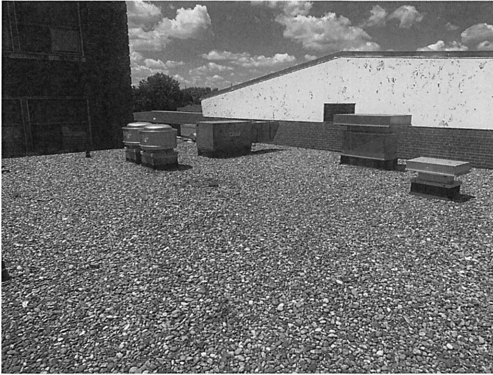
View from on the kitchen roof.
