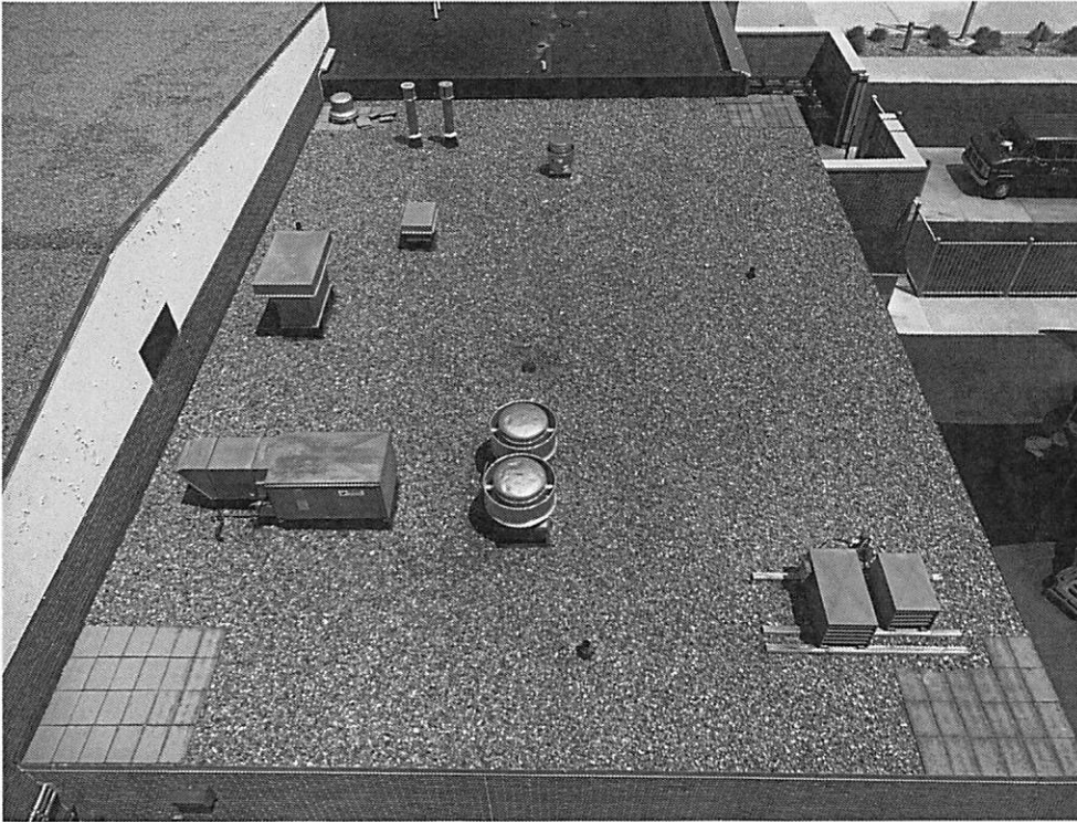
Kitchen roof shown from above.
