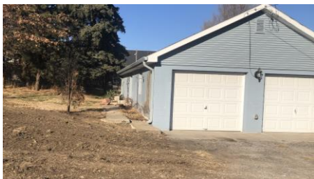
Area for water hydrant
