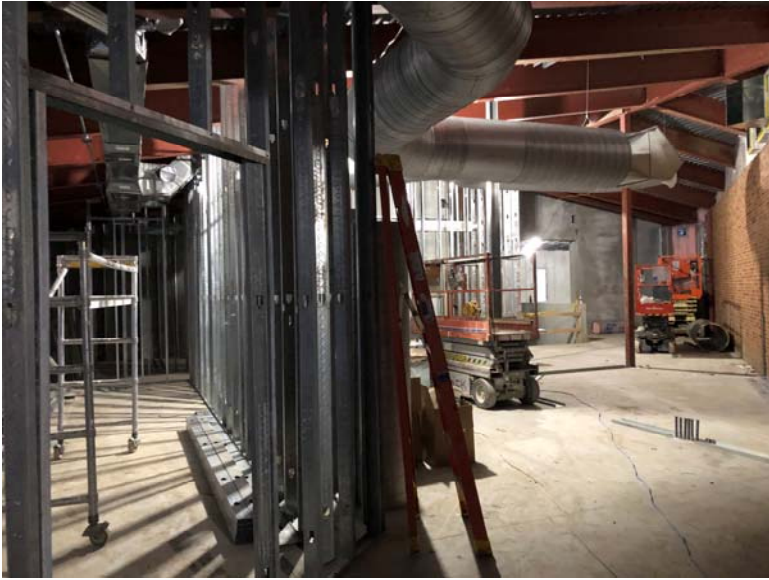
Commons light gauge framing at women's restroom
