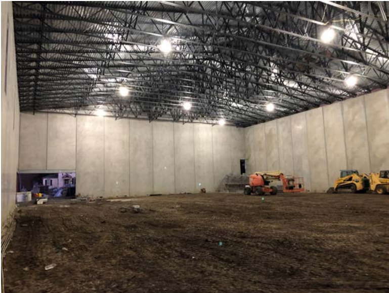
Gymnasium interior looking east
