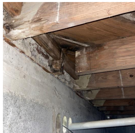
Photo #30 Typical joist connection at foundation wall at northwest elevation.
