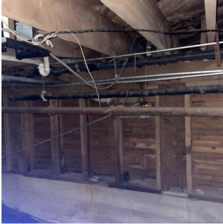
Photo #13 Wood framed wall in crawlspace near basement entrance.
