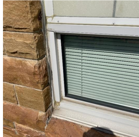
Photo #2 Typical window condition. Sealant noted at frame.
