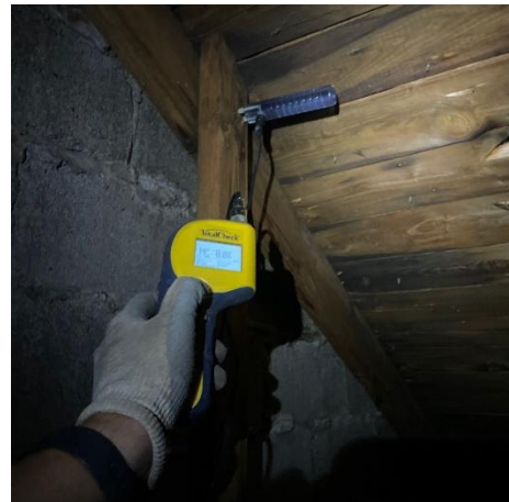
Photo #40 Typical moisture probe of wood framing in attic.
