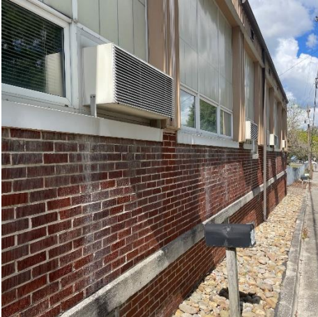
Photo #7 HVAC units and some staining at brick at northeast elevation.
