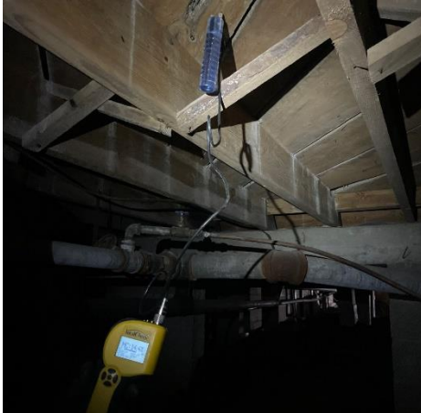
Photo #19 Typical moisture probe of floor diaphragm boards.
