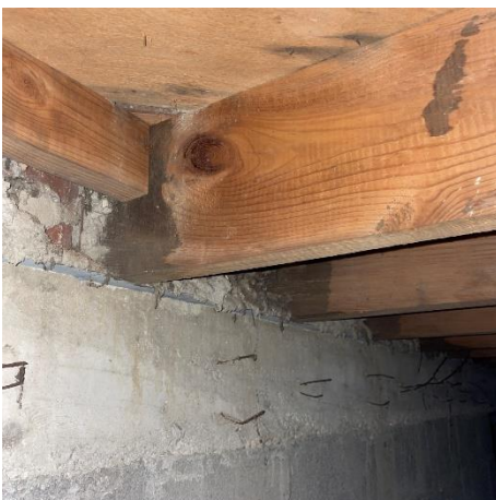
Photo #23 Typical joist connection at perimeter foundation.
