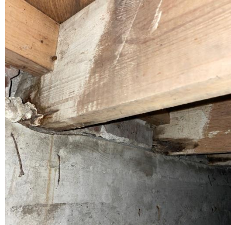
Photo #26 Joist connection at perimeter foundation at northwest elevation, near sample #2.
