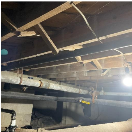
Photo #9 Typical crawlspace condition.
