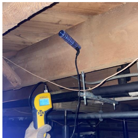
Photo #16 Typical moisture probe measure probe of crawlspace floor joists.
