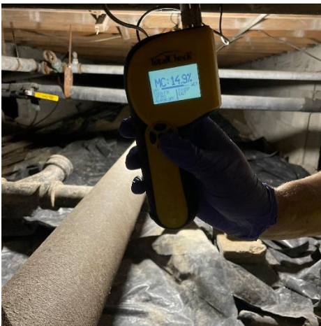
Photo #17 Typical moisture probe measurement.
