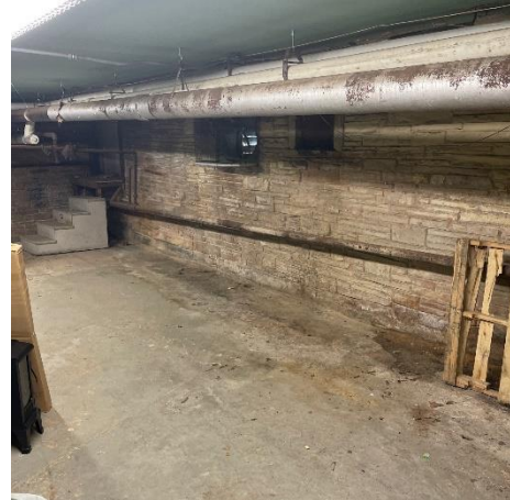
Photo #8 Basement exterior wall, northeast elevation.
