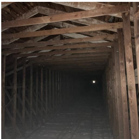
Photo #35 Typical wing of building in attic.
