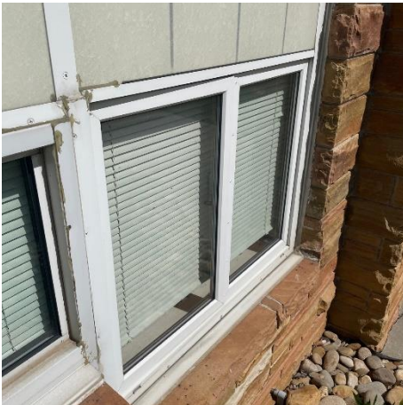
Photo #3 Typical window condition, sealant noted at frame.
