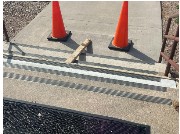
Repaired back step
