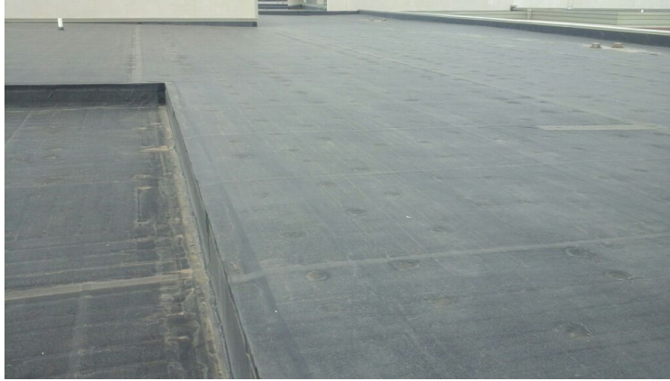
Photo showing overview of Area 01 Roof.
