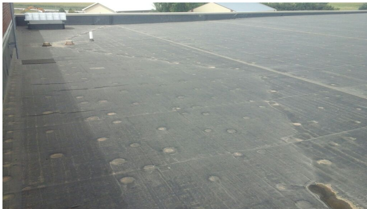
Photo showing additional overview of Area 13 Roof.
