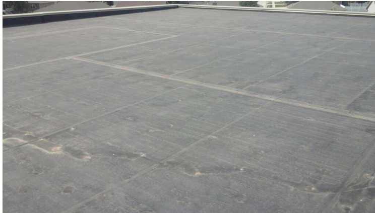
Photo showing overview of Area 05 Roof.
