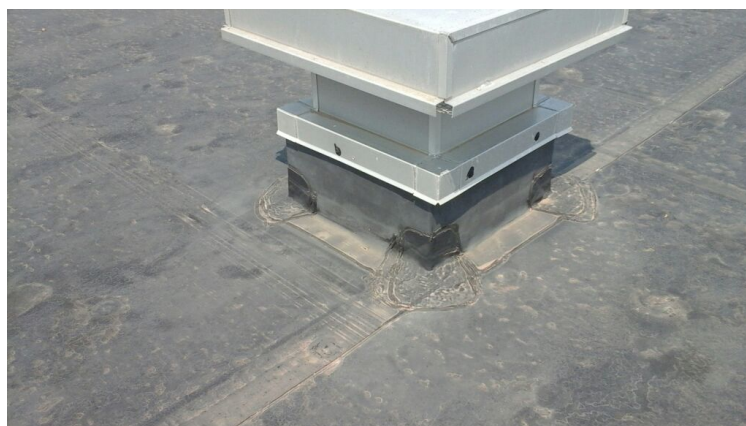
Photo showing condition of projection flashings.
