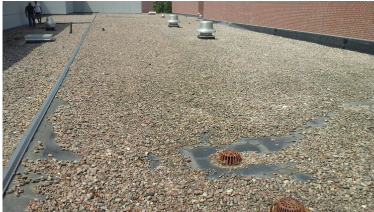
Photo showing additional overview of Area 10 Roof.
