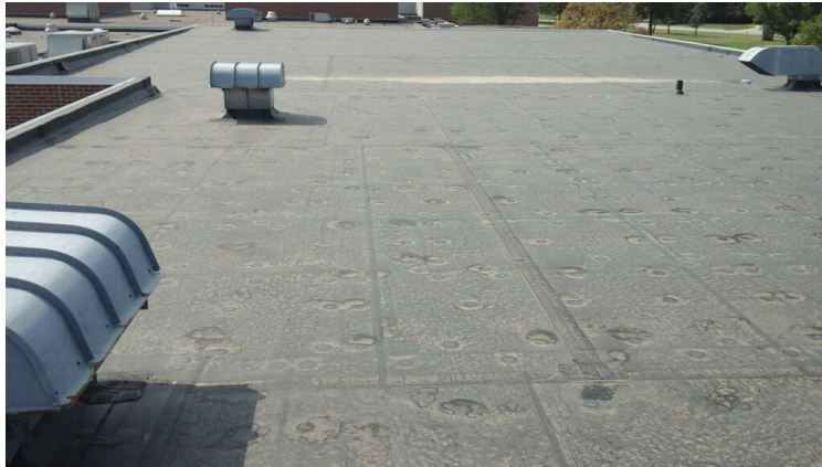
Photo showing overview of Area 01 Roof.
