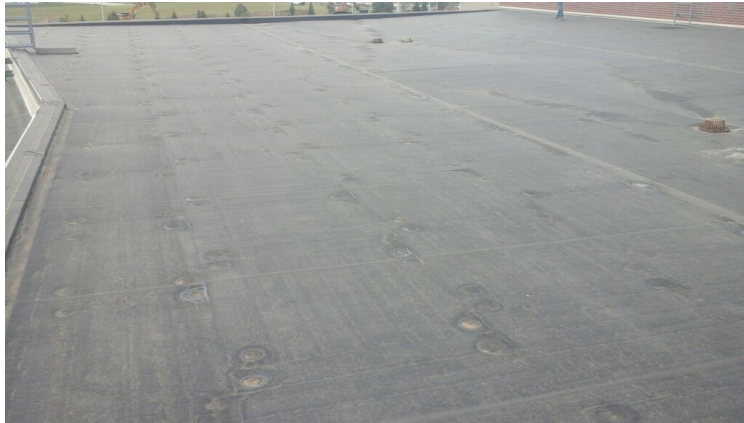
Photo showing overview of Area 11 Roof.
