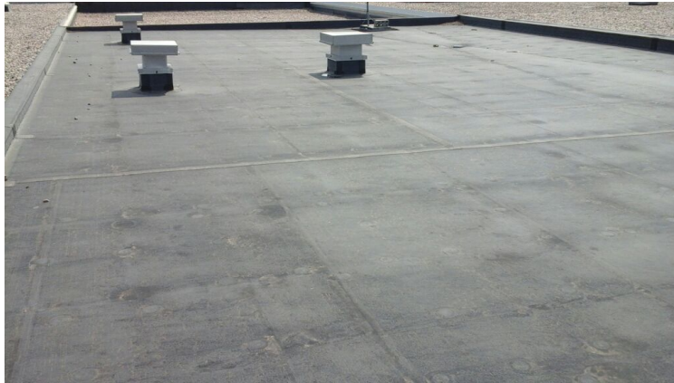
Photo showing overview of Area 07 Roof.
