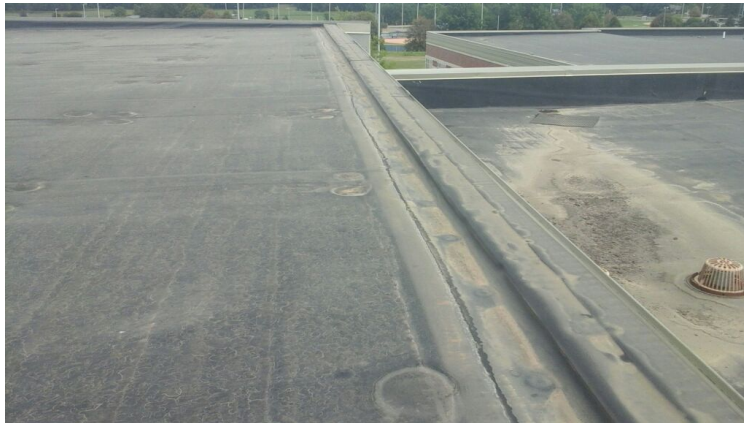
Photo showing condition of the form flashings.
