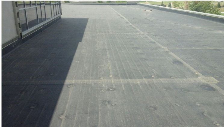
Photo showing overview of Area 06 Roof.
