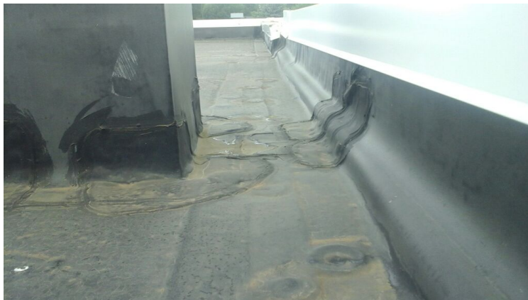
Photo showing condition of the perimeter flashings.
