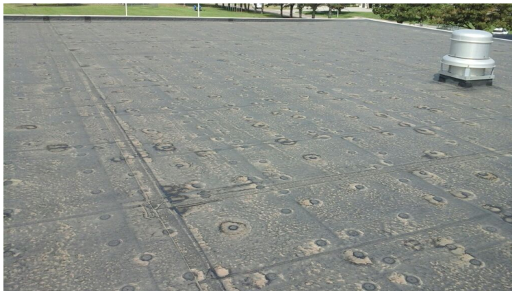
Photo showing additional overview of Area 01 Roof.
