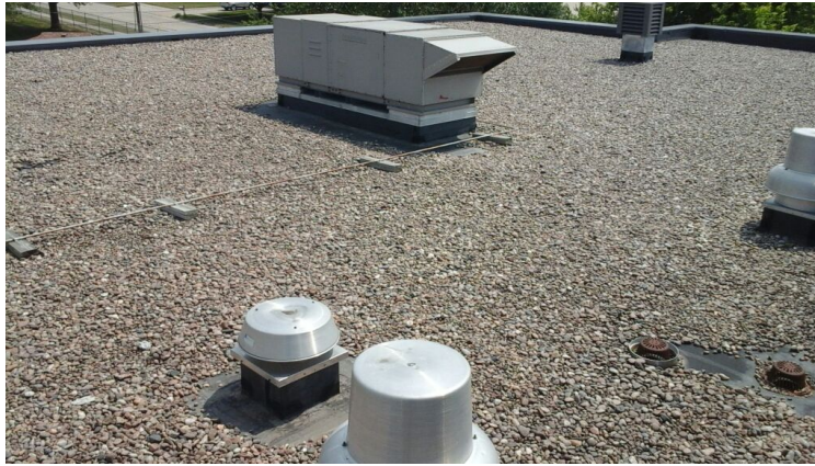
Photo showing overview of Area 21 Roof.
