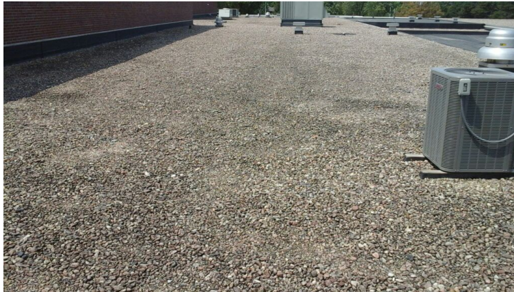
Photo showing overview of Area 10 Roof.
