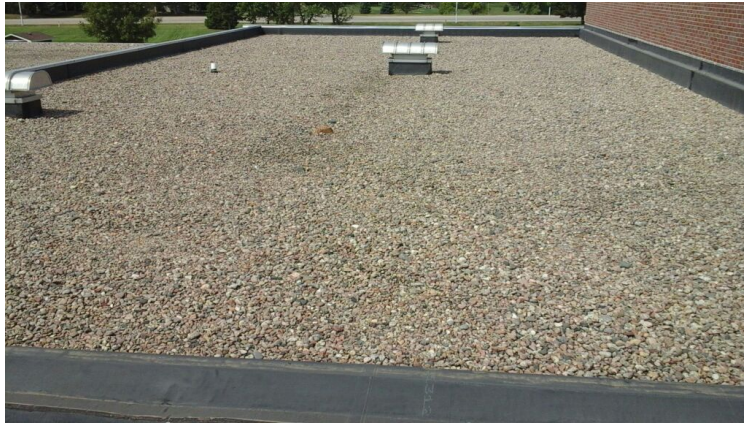
Photo showing overview of Area 03 Roof.
