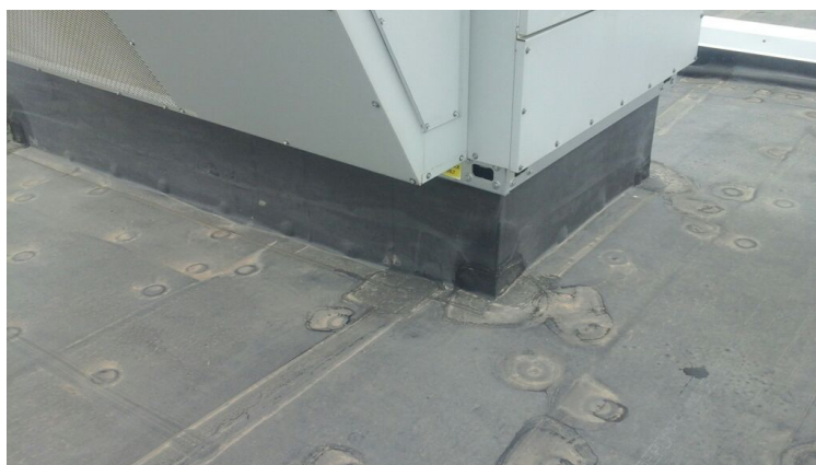
Photo showing condition of projection flashings.
