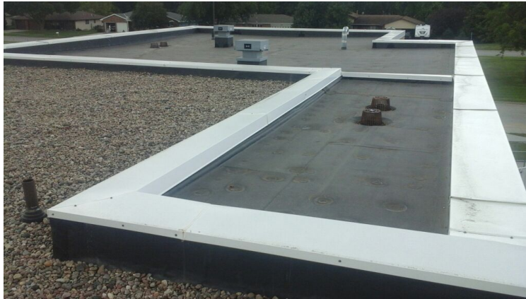
Photo showing overview of Area 07 Roof.
