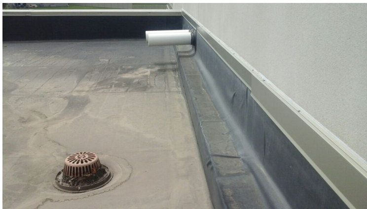
Photo showing condition of the perimeter flashings.
