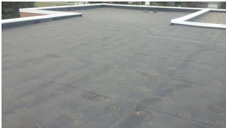
Photo showing additional overview of Area 08 Roof.
