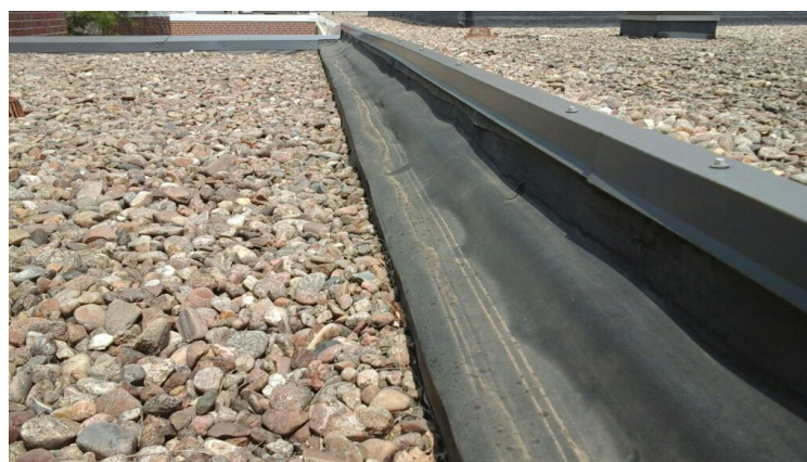
Photo showing condition of the expansion joint.
