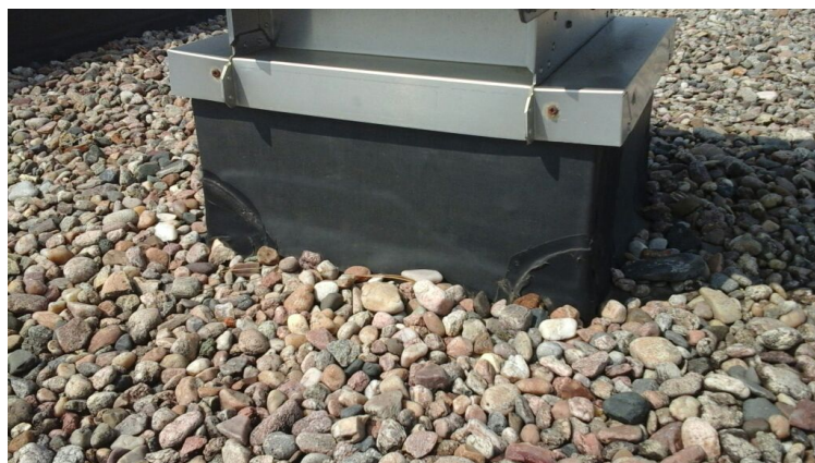
Photo showing condition of projection flashings.
