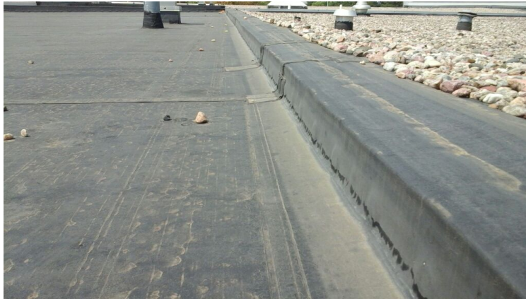
Photo showing condition of the perimeter flashings.
