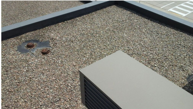
Photo showing overview of Area 16 Roof.
