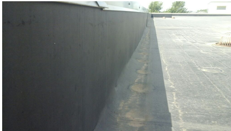
Photo showing condition of the perimeter flashings.
