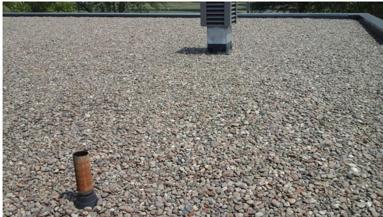
Photo showing additional overview of Area 21 Roof.
