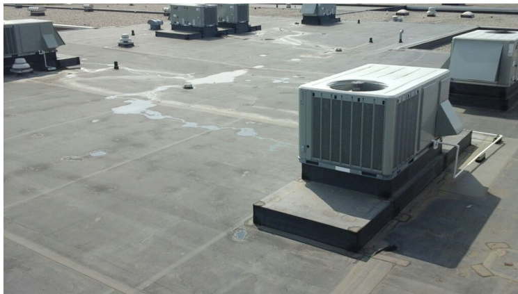
Photo showing additional overview of Area 02 Roof.
