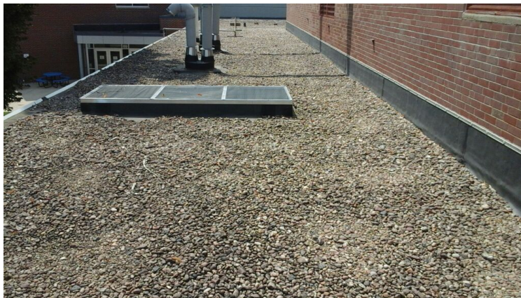
Photo showing additional overview of Area 10 Roof.
