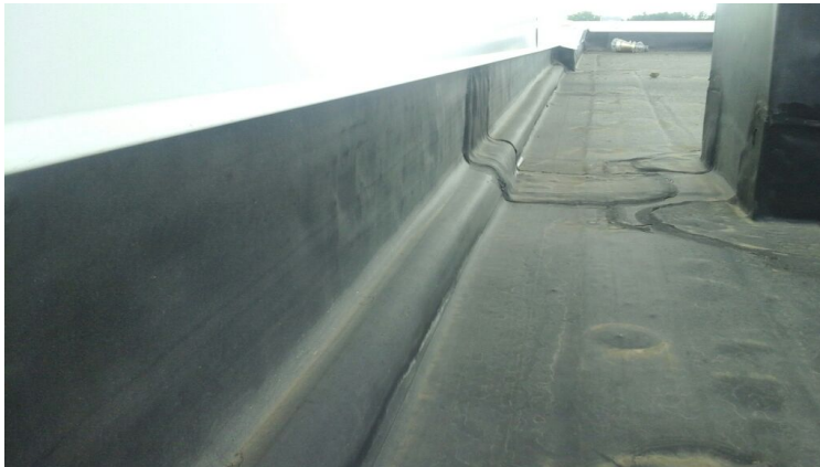
Photo showing condition of the perimeter flashings.
