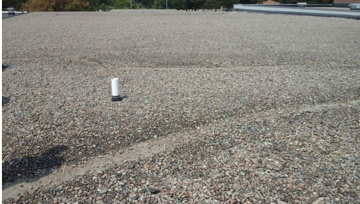
Photo showing overview of Area 06 Roof.
