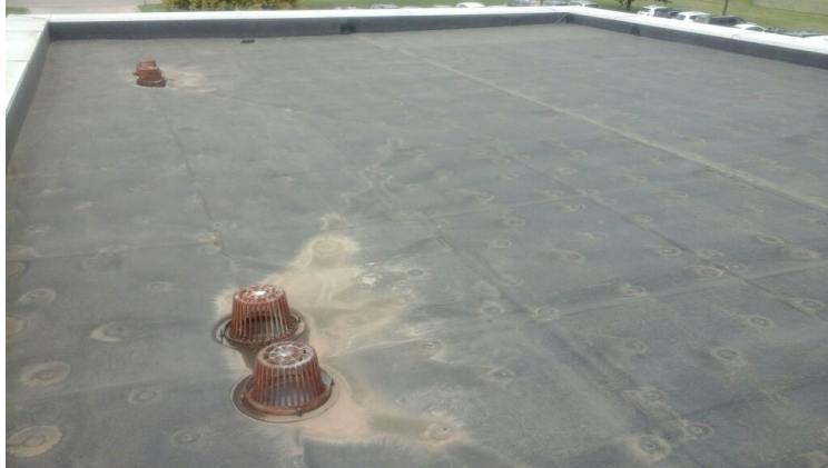
Photo showing overview of Area 01 Roof.
