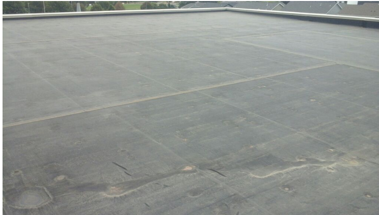
Photo showing overview of Area 04 Roof.
