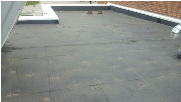
Photo showing additional overview of Area 02 Roof.
