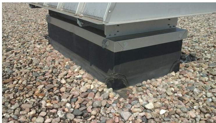
Photo showing condition of projection flashings.
