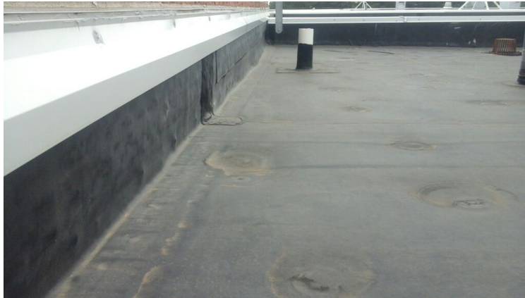
Photo showing condition of the perimeter flashings.
