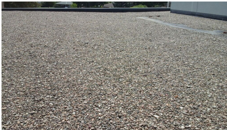
Photo showing additional overview of Area 17 Roof.
