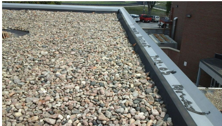
Photo showing condition of perimeter flashings.
