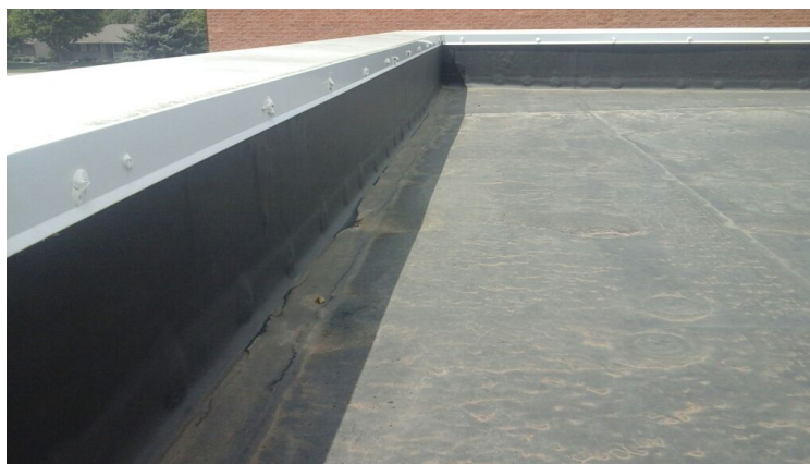
Photo showing condition of the perimeter flashings.
