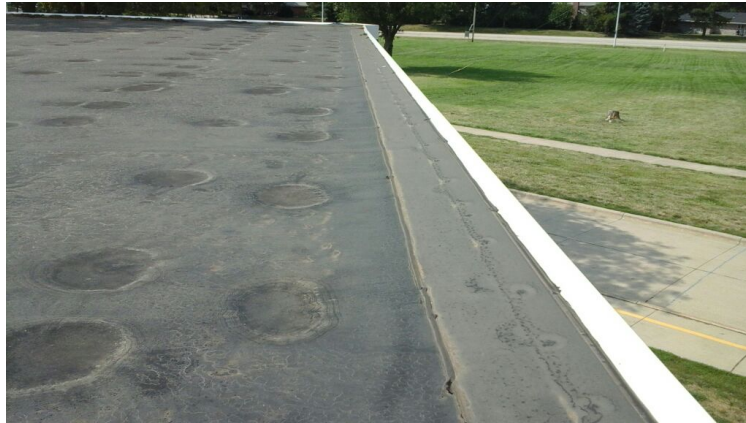
Photo showing condition of the form flashings.
