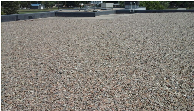
Photo showing additional overview of Area 20 Roof.
