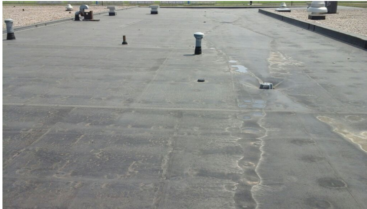
Photo showing overview of Area 09 Roof.
