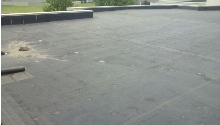
Photo showing overview of Area 02 Roof.
