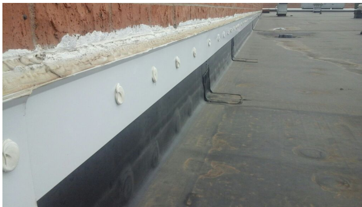
Photo showing condition of the perimeter flashings.
