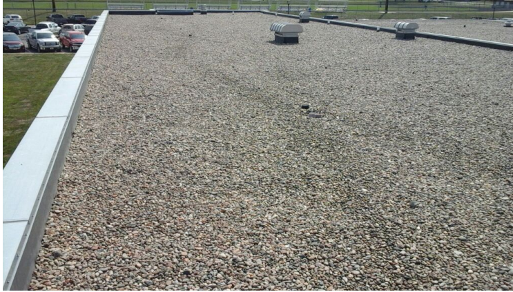
Photo showing overview of Area 04 Roof.
