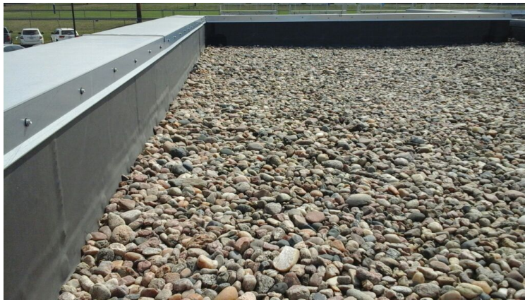
Photo showing condition of the perimeter flashings.
