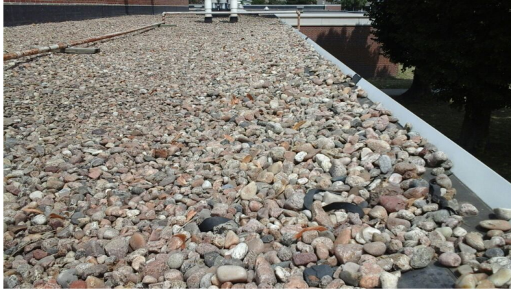
Photo showing condition of the form flashings.
