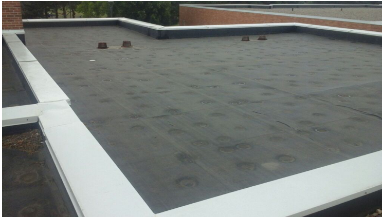
Photo showing overview of Area 04 Roof.
