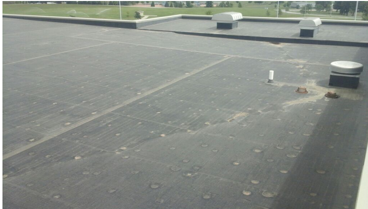
Photo showing overview of Area 13 Roof.
