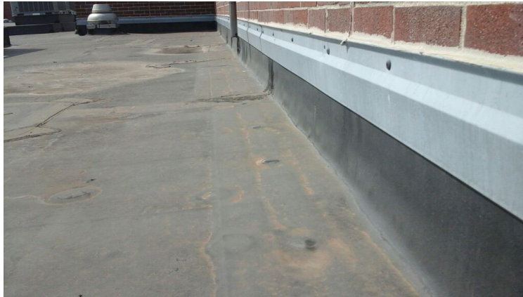
Photo showing condition of the perimeter flashings.
