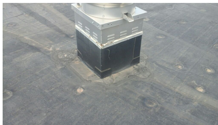
Photo showing condition of projection flashings.
