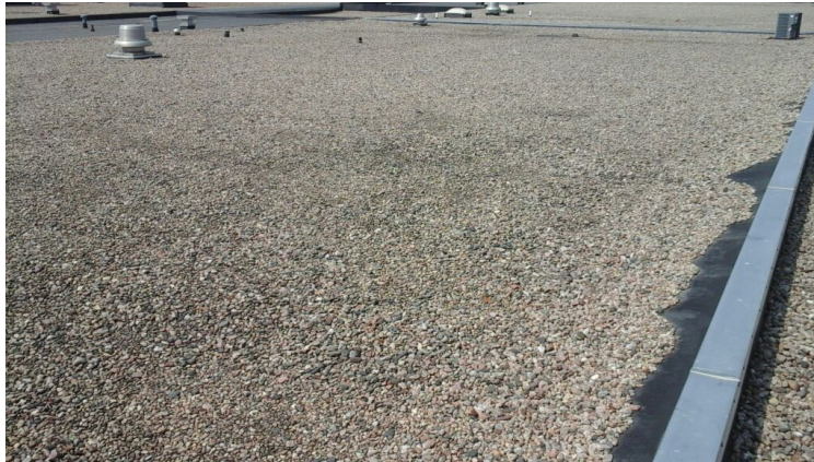
Photo showing overview of Area 05 Roof.
