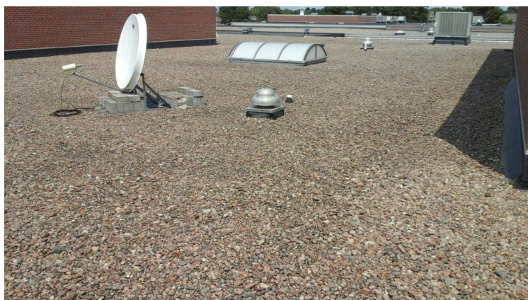
Photo showing additional overview of Area 10 Roof.
