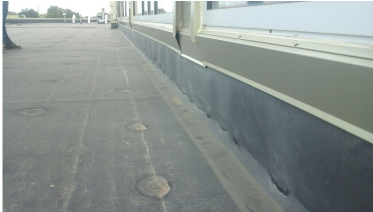
Photo showing condition of the counter flashing along the window wall.
