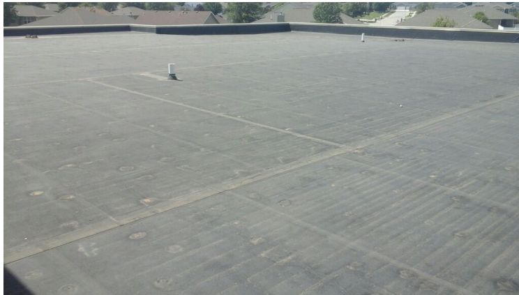
Photo showing additional overview of Area 06 Roof.
