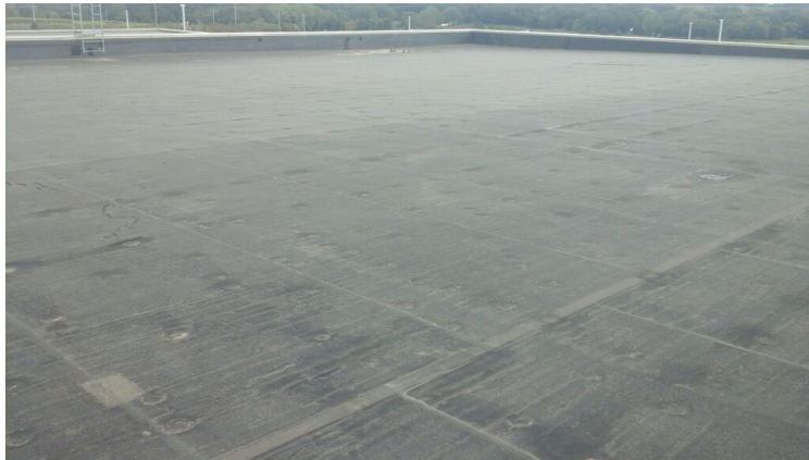
Photo showing overview of Area 12 Roof.
