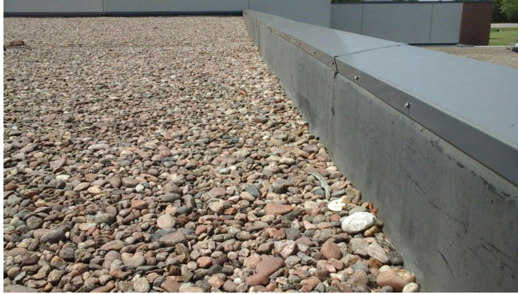
Photo showing condition of the perimeter flashings.
