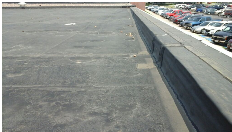
Photo showing condition of the form flashings.
