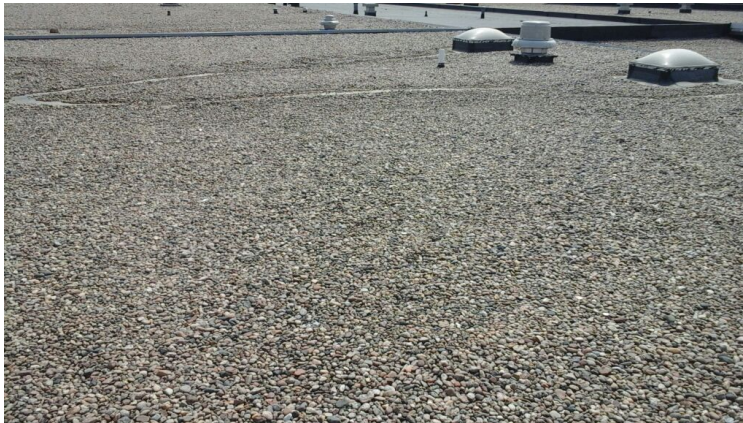
Photo showing additional overview of Area 06.
