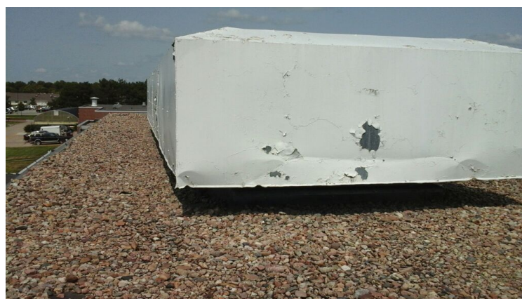
Photo showing condition of projection.
