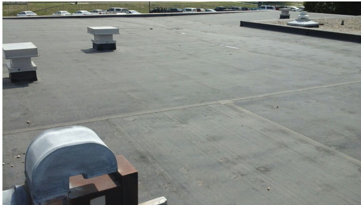
Photo showing additional overview of Area 09 Roof.
