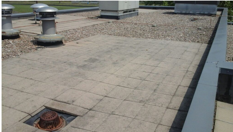
Photo showing overview of Area 22 roof.
