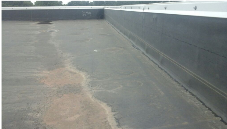
Photo showing condition of the perimeter flashings.
