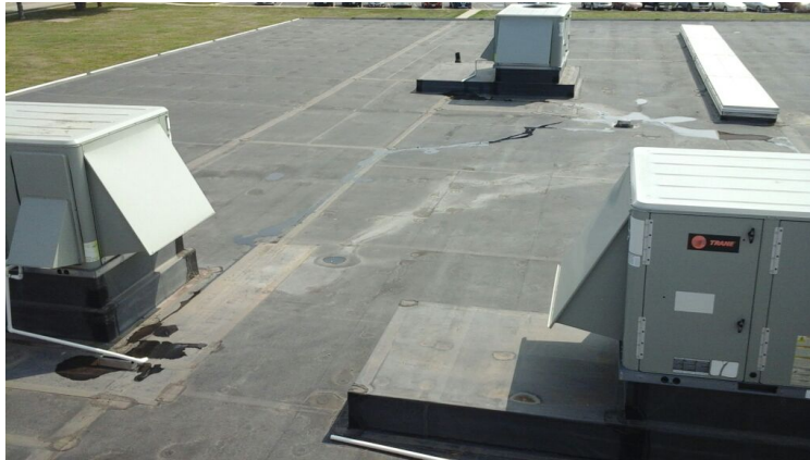
Photo showing overview of Area 02 Roof.
