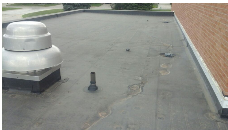
Photo showing additional overview of Area 03 Roof.
