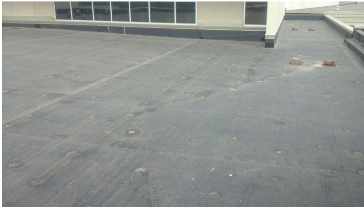
Photo showing additional overview of Area 02 Roof.
