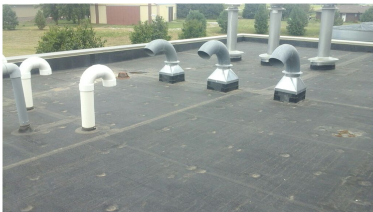
Photo showing condition of the projection flashings.
