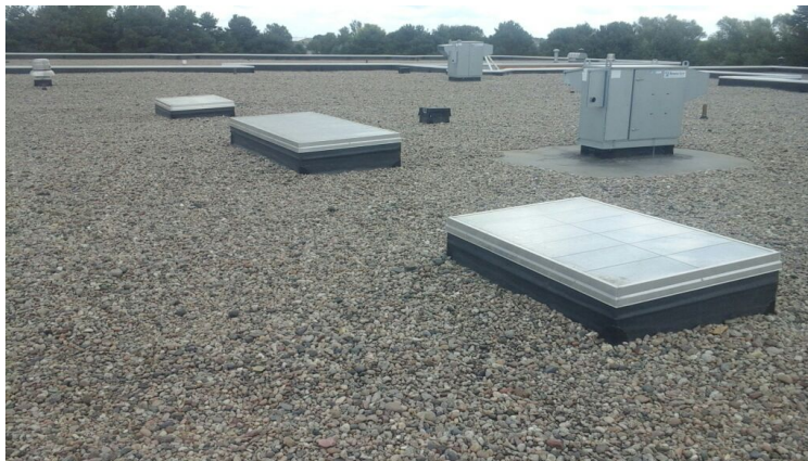
Photo showing condition of the skylights.
