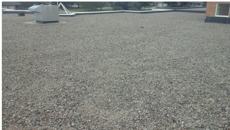
Photo showing additional overview of Area 05 Roof.
