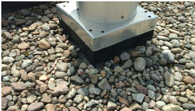
Photo showing condition of projection flashings.
