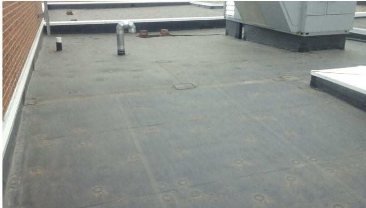
Photo showing overview of Area 02 Roof.
