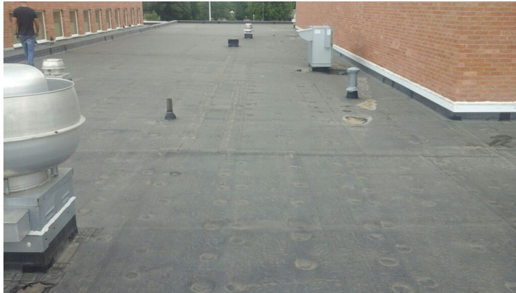
Photo showing overview of Area 03 Roof.
