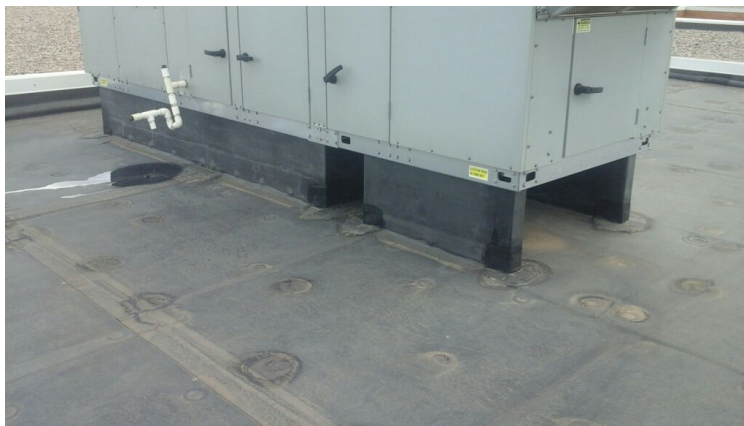
Photo showing condition of projection flashings.
