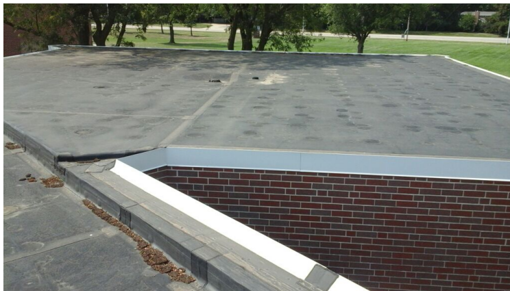
Photo showing additional overview of Area 07 Roof.
