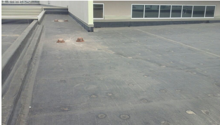
Photo showing additional overview of Area 02 Roof.
