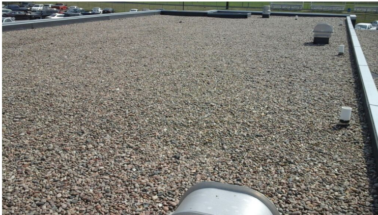
Photo showing additional overview of Area 04 Roof.
