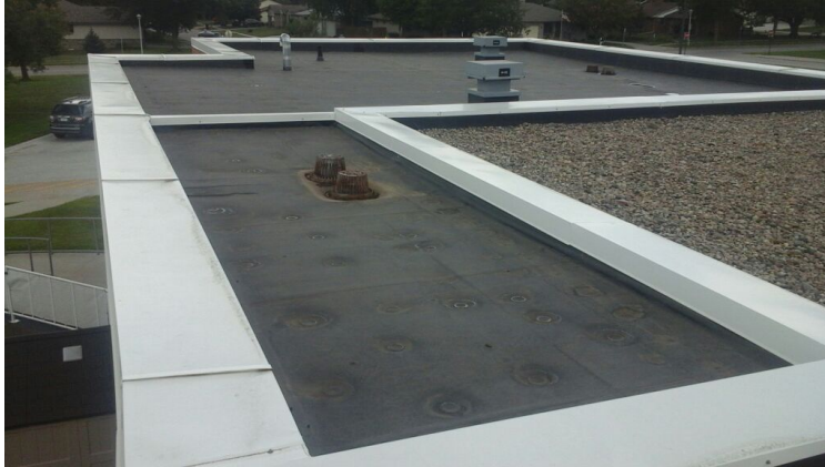
Photo showing overview of Area 06 Roof.
