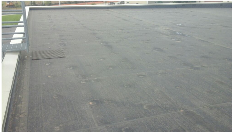
Photo showing overview of Area 12 Roof.
