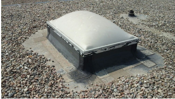
Photo showing condition of the skylights.
