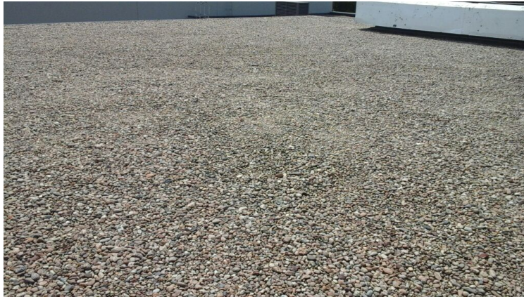
Photo showing overview of Area 23 Roof.
