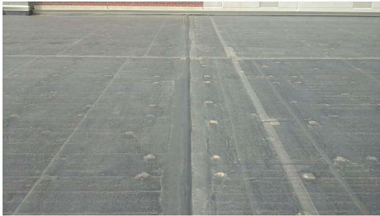
Photoshowing condition of the expansion joint.
