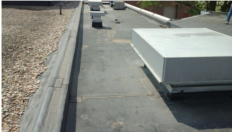
Photo showing additional overview of Area 07 Roof.
