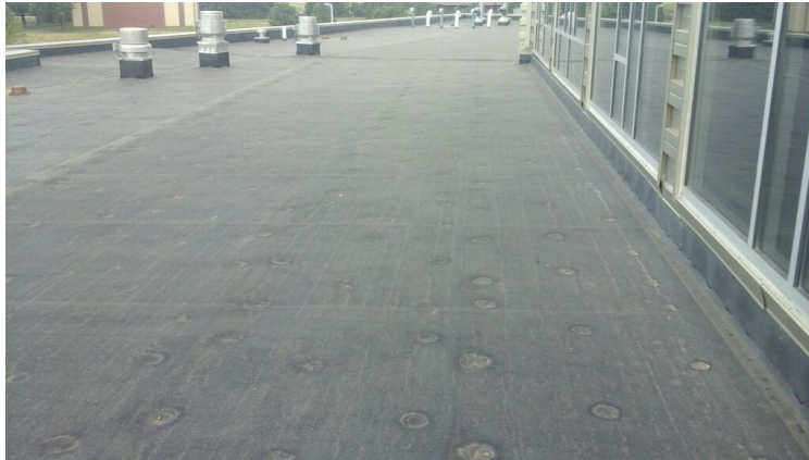
Photo showing overview of Area 08 Roof.
