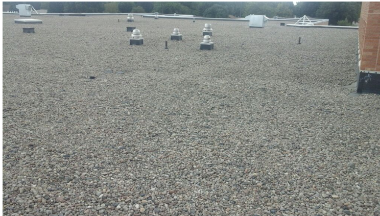
Photo showing additional overview of Area 05 Roof.
