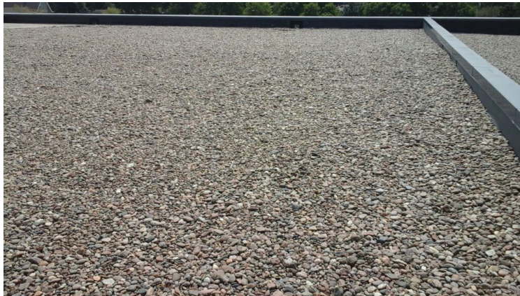
Photo showing additional overview of Area 15 Roof.
