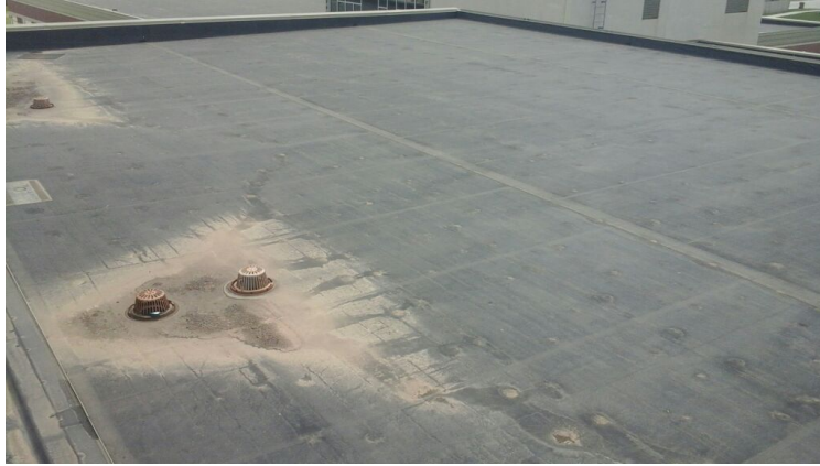
Photo showing overview of Area 09 Roof.
