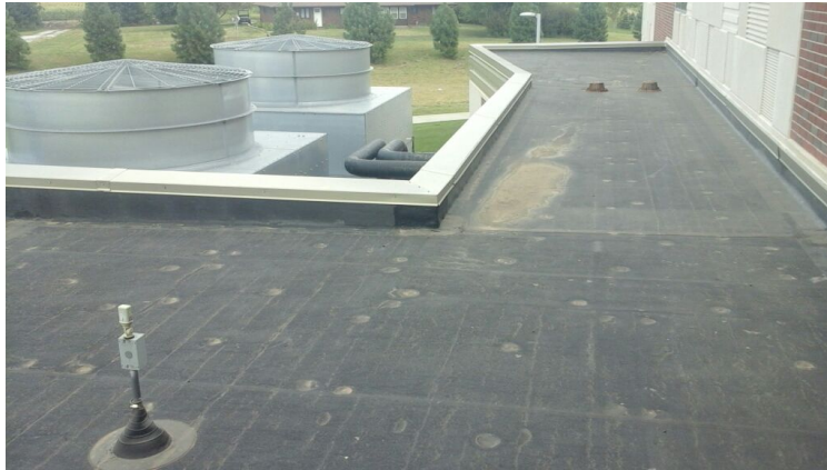
Photo showing additional overview of Area 08 Roof.
