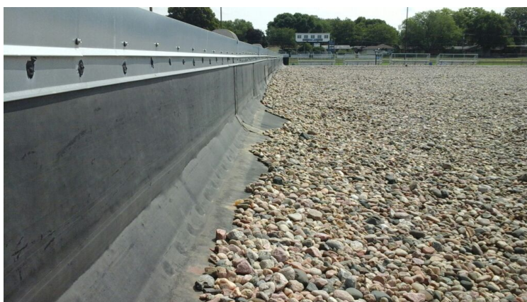
Photo showing condition of the perimeter flashings.
