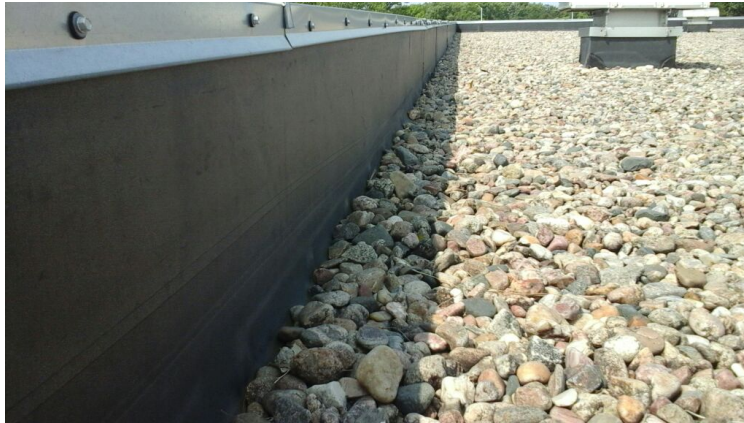
Photo showing condition of the perimeter flashings.
