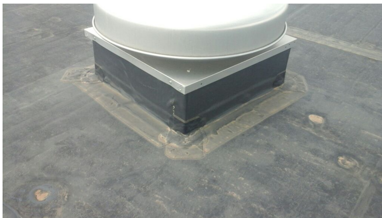
Photo showing condition of projection flashings.
