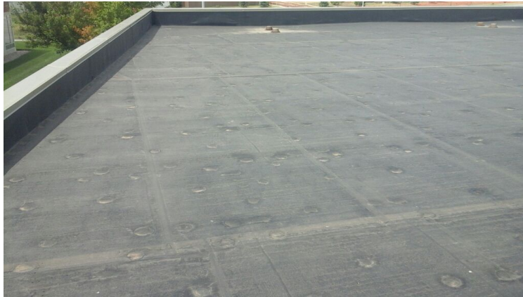
Photo showing overview of Area 07 Roof.
