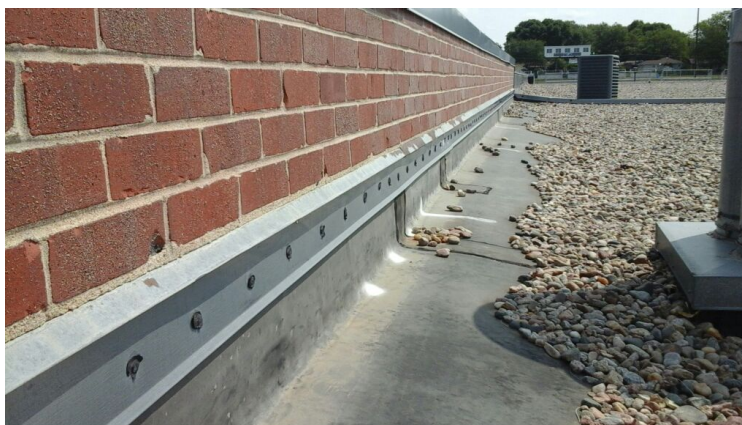
Photo showing condition of the perimeter flashings.
