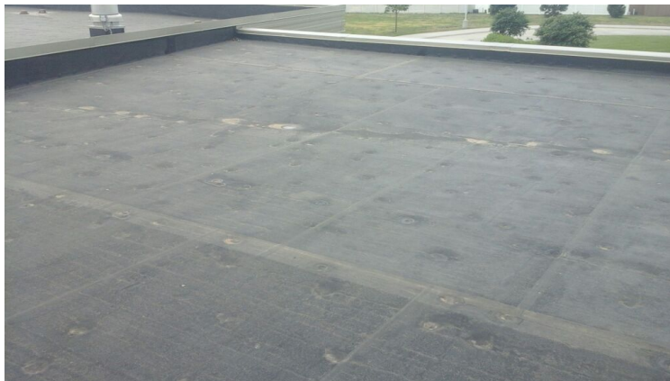
Photo showing additional overview of Area 08 Roof.
