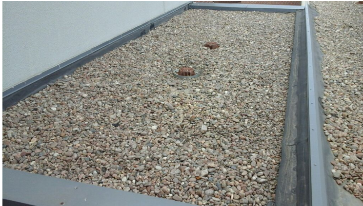
Photo showing overview of Area 12 Roof.
