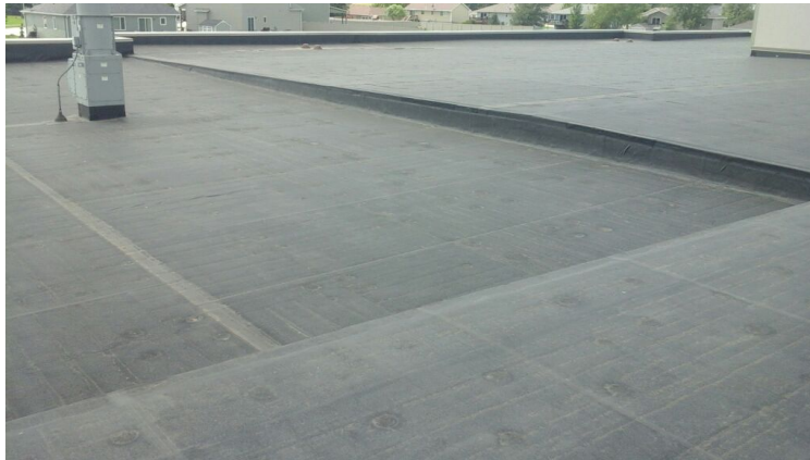
Photo showing additional overview of Area 01 Roof.
