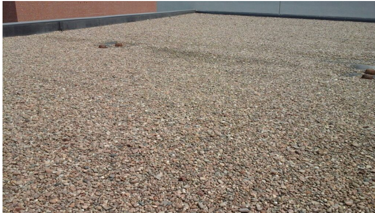
Photo showing overview of Area 17 Roof.
