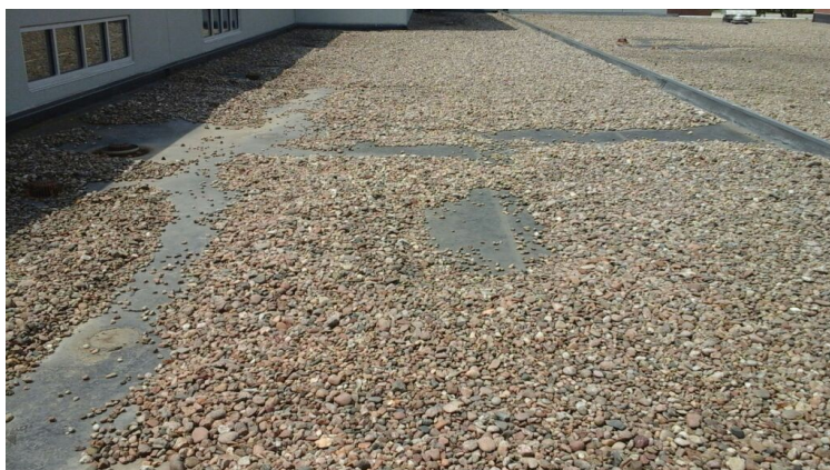
Photo showing additional overview of Area 11 Roof.
