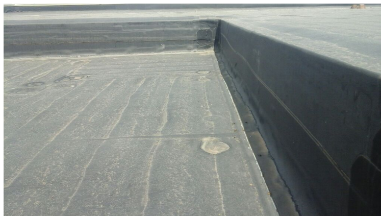
Photo showing condition of the interior flashings.
