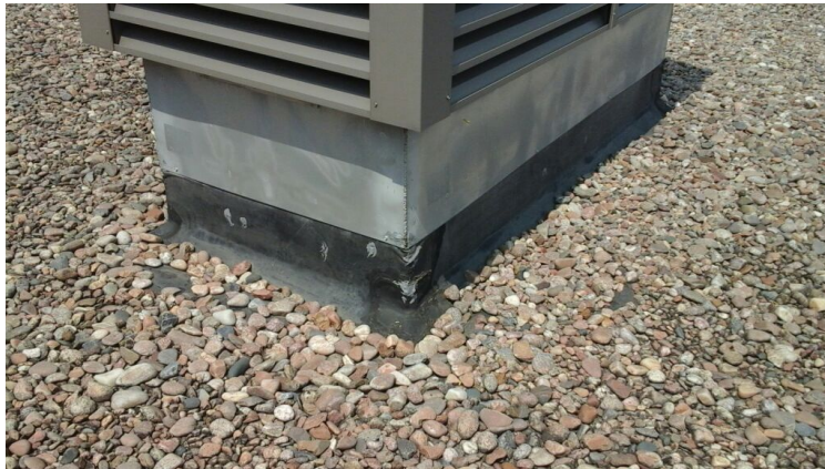
Photo showing condition of projection flashings.
