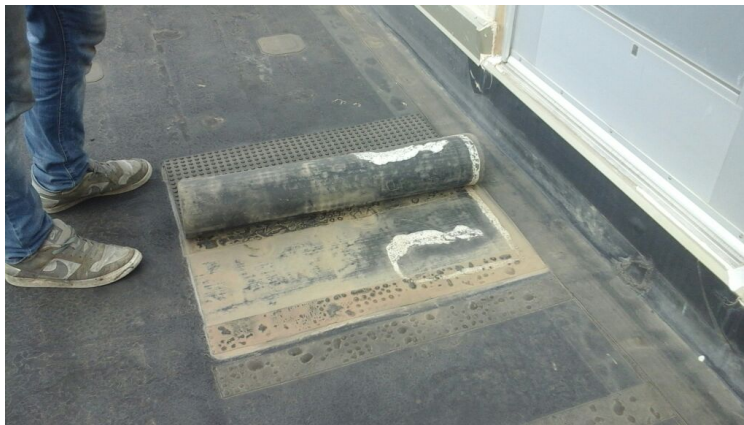
Photo showing walk pad pulling up at door.
