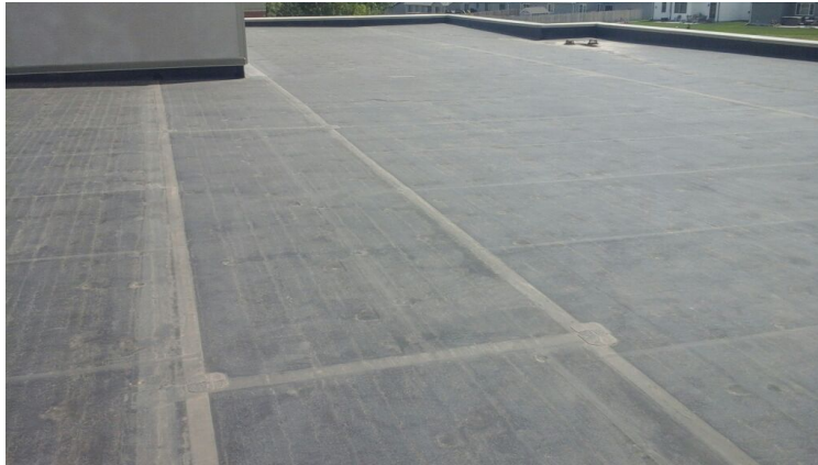
Photo showing additional overview of Area 06 Roof.
