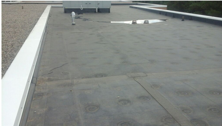
Photo showing overview of Area 08 Roof.
