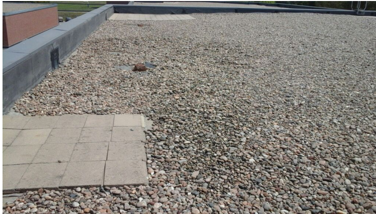
Photo showing overview of Area 15 Roof.
