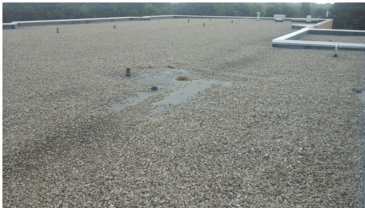
Photo showing additional overview of Area 09 Roof.
