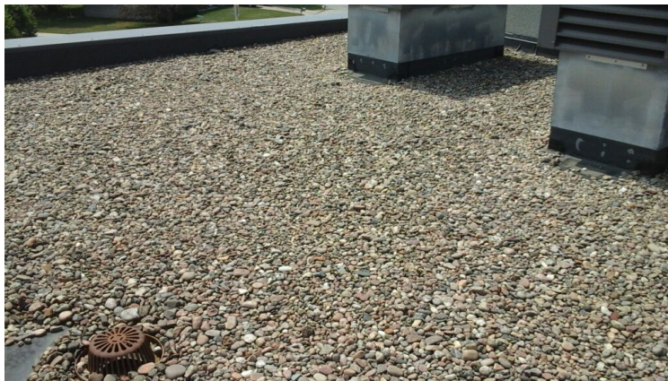
Photo showing additional overview of Area 16 Roof.
