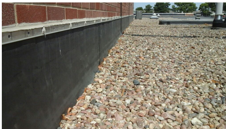
Photo showing condition of the perimeter flashings.
