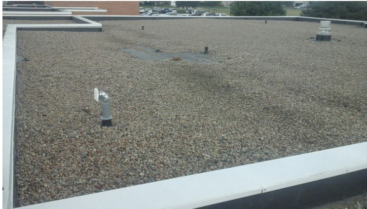
Photo showing overview of Area 09 Roof.
