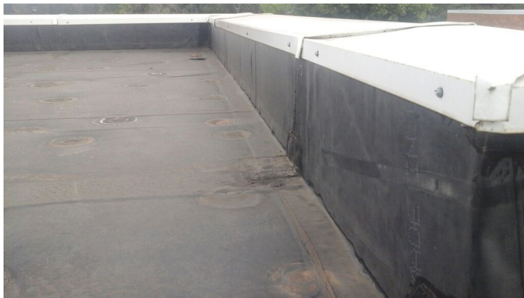
Photo showing condition of the perimeter flashings.
