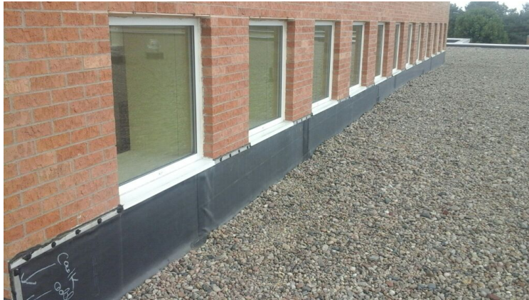
Photo showing condition of the perimeter flashings along the window wall.
