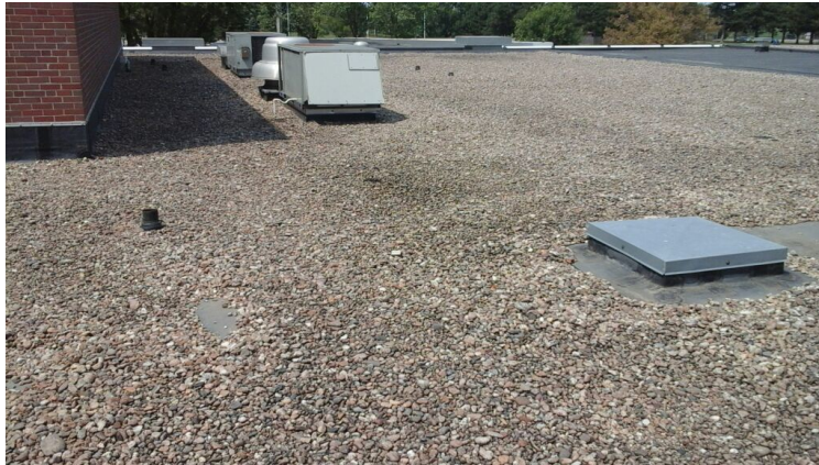
Photo showing additional overview of Area 10 Roof.
