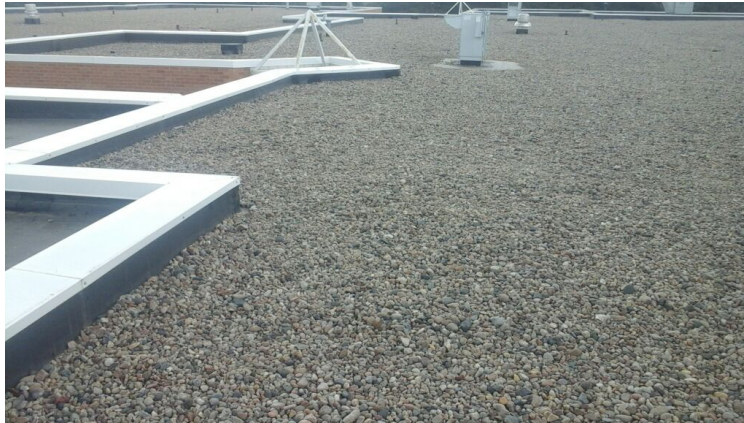
Photo showing overview of Area 05 Roof.
