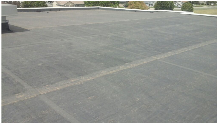
Photo showing additional overview of Area 10 Roof.
