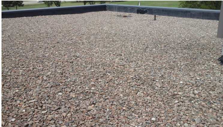
Photo showing overview of Area 13 Roof.
