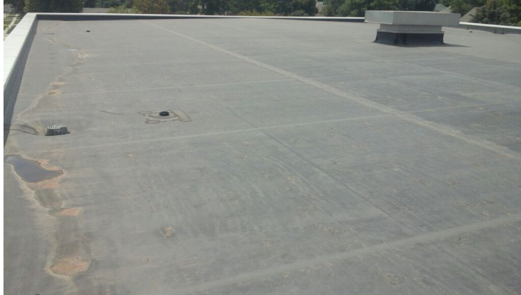
Photo showing overview of Area 10 Roof.
