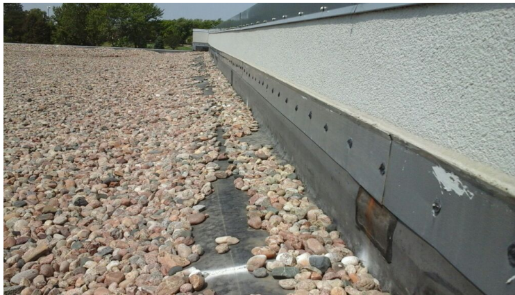
Photo showing condition of the perimeter flashings.
