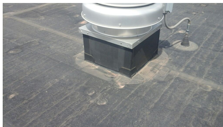
Photo showing condition of projection flashings.
