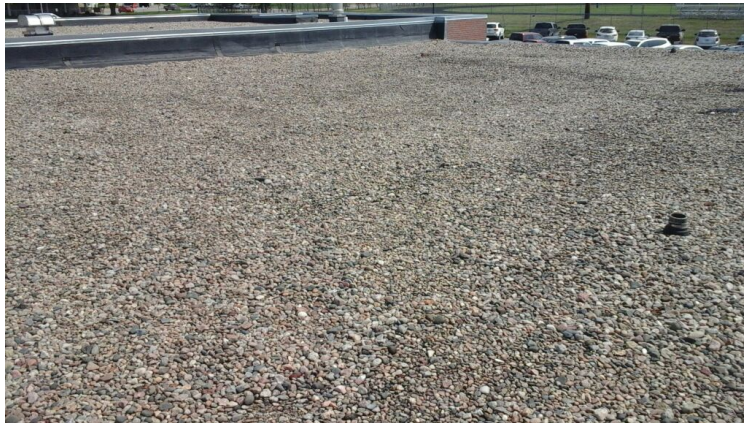
Photo showing additional overview of Area 05 Roof.
