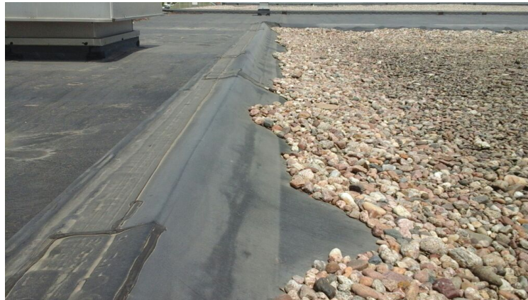
Photo showing condition of expansion joint.
