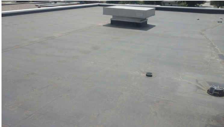
Photo showing overview of Area 11.
