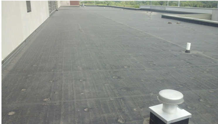
Photo showing overview of Area 03 Roof.
