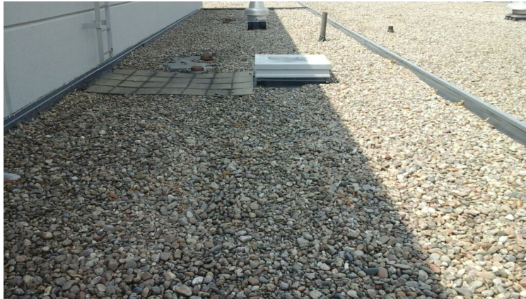
Photo showing overview of Area 11 Roof.
