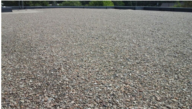
Photo showing overview of Area 20 Roof.
