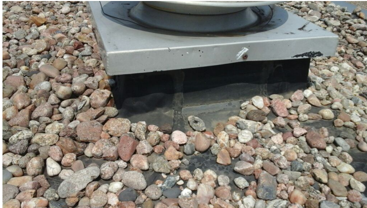
Photo showing condition of projection flashings.
