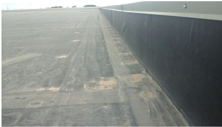
Photo showing condition of the perimeter flashings.
