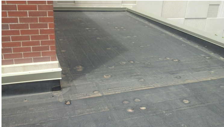
Photo showing additional overview of Area 03 Roof.
