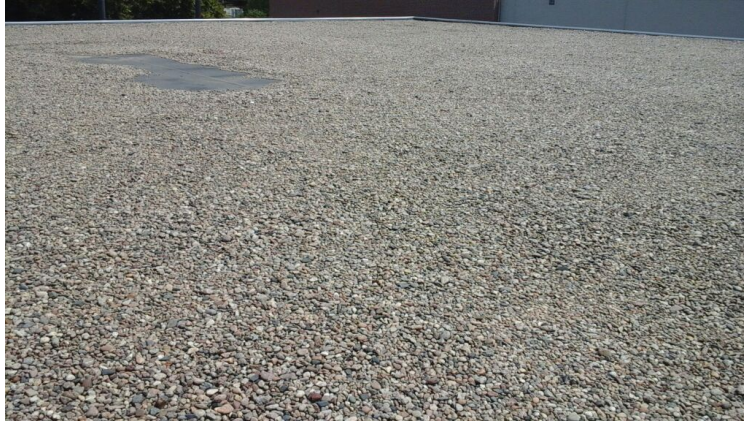
Photo showing overview of Area 24 roof.
