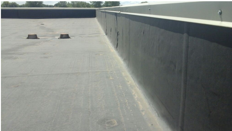
Photo showing condition of the perimeter flashings.
