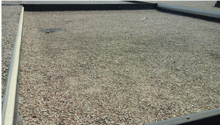
Photo showing overview of 08 Roof.
