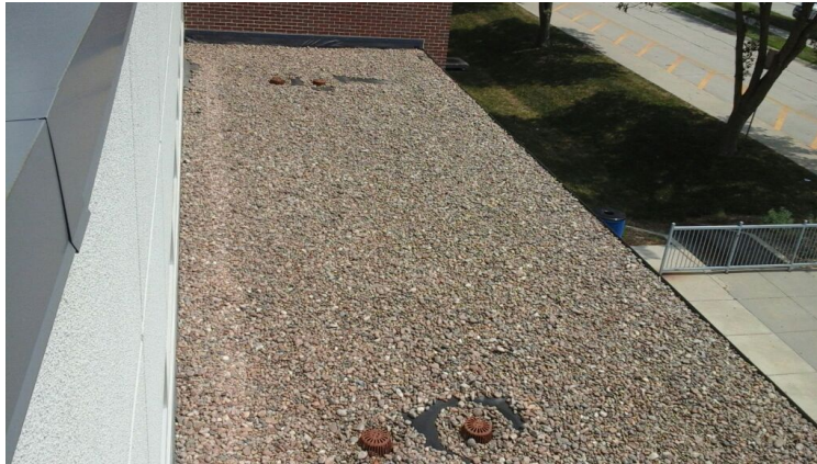
Photo showing overview of Area 19 Roof.
