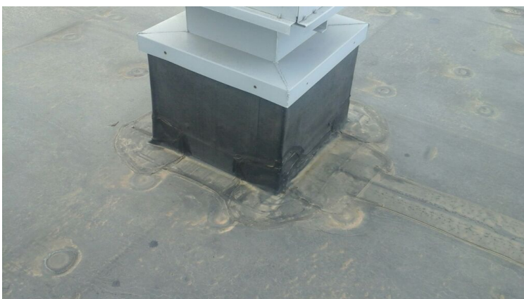
Photo showing condition of projection flashings.
