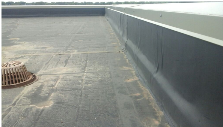
Photo showing condition of the perimeter flashings.
