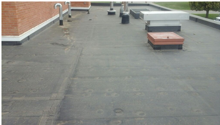
Photo showing additional overview of Area 03 Roof.
