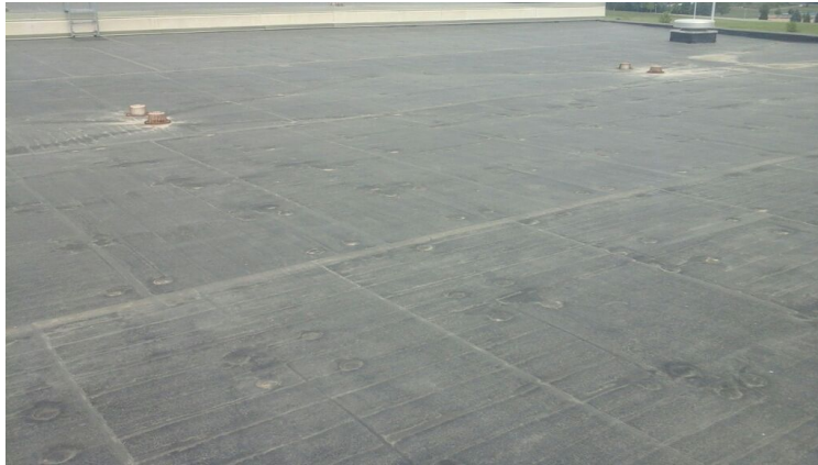
Photo showing overview of Area 10 Roof.
