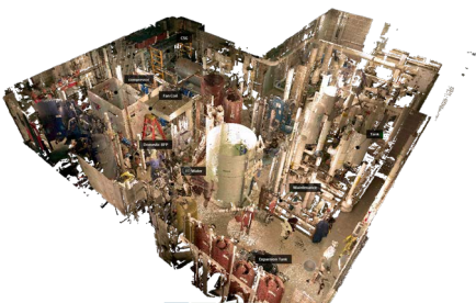
Point Cloud Scan of Existing Equipment Room
